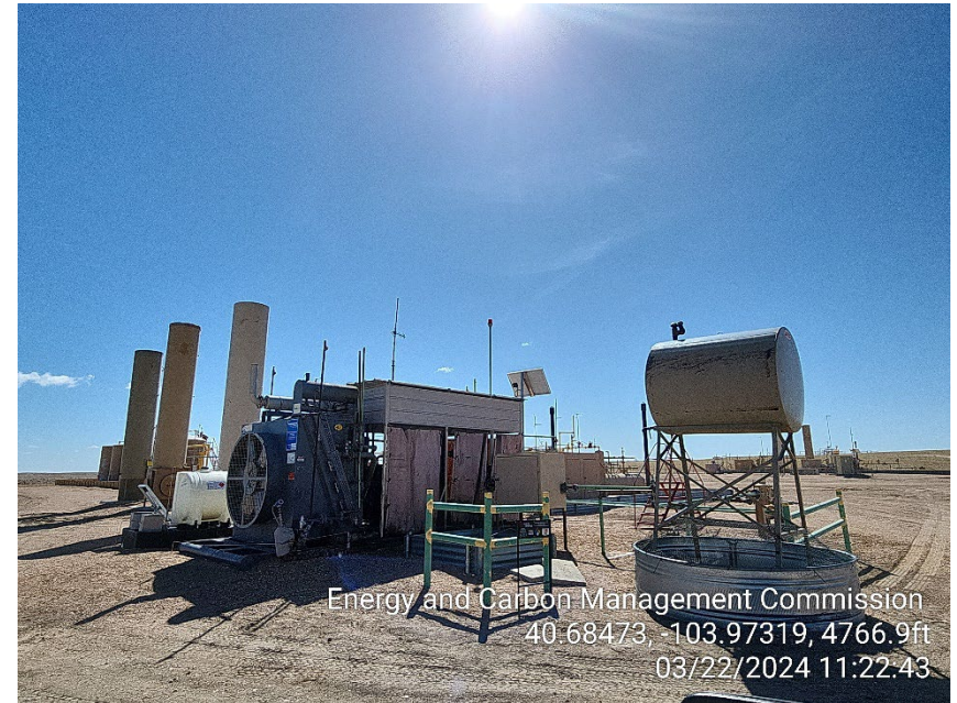
Photo 2 – ECDs and Compressor
