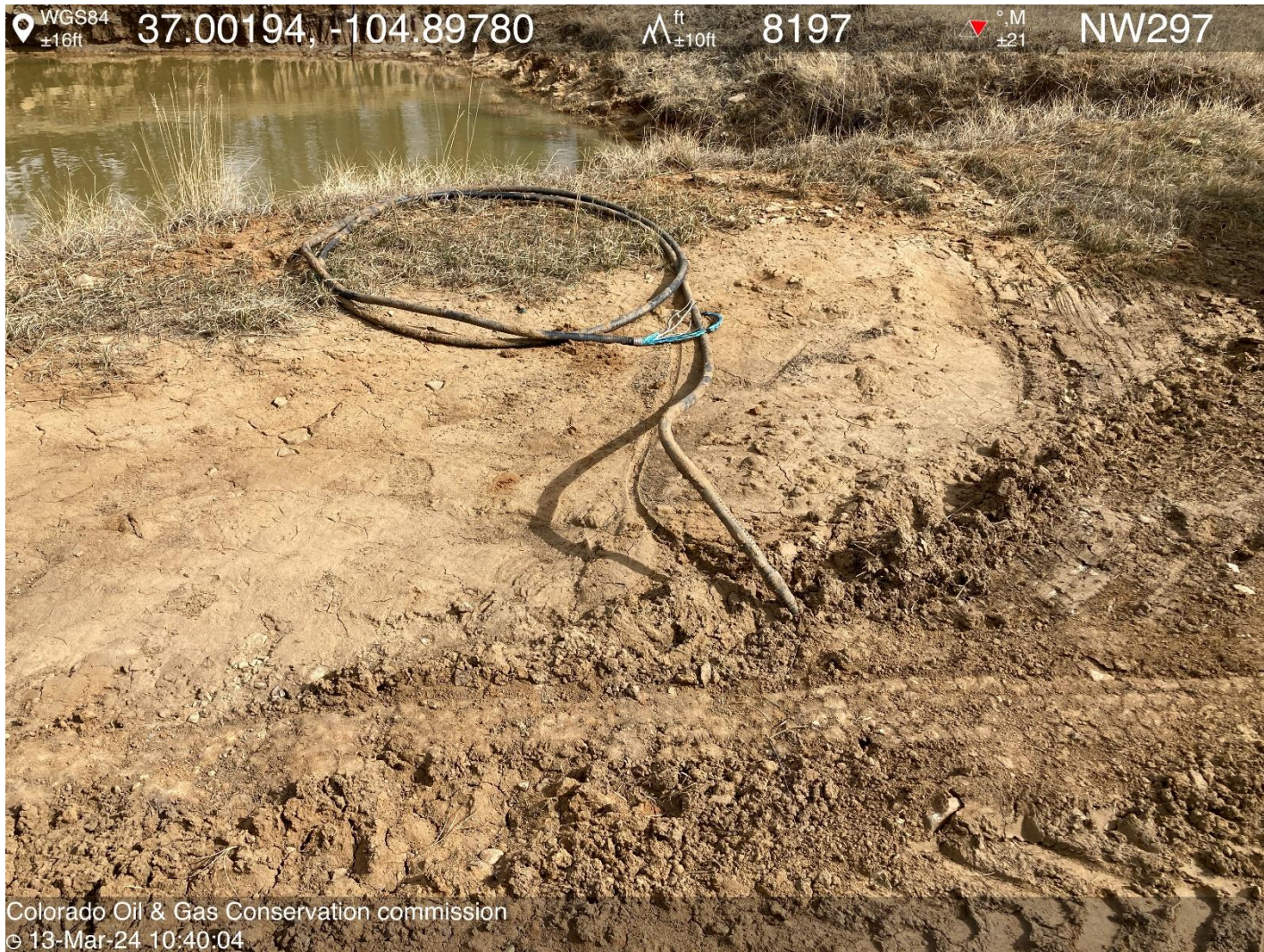
PHOTO 4: UNUSED EQUIPMENT (ELECTRIC LINE COMING OUT OF THE GROUND BETWEEN METER HOUSE AND WELLHEAD). REMOVE UNUSED EQUIPMENT PER RULE 606. CA DATE 4-26-2024.
