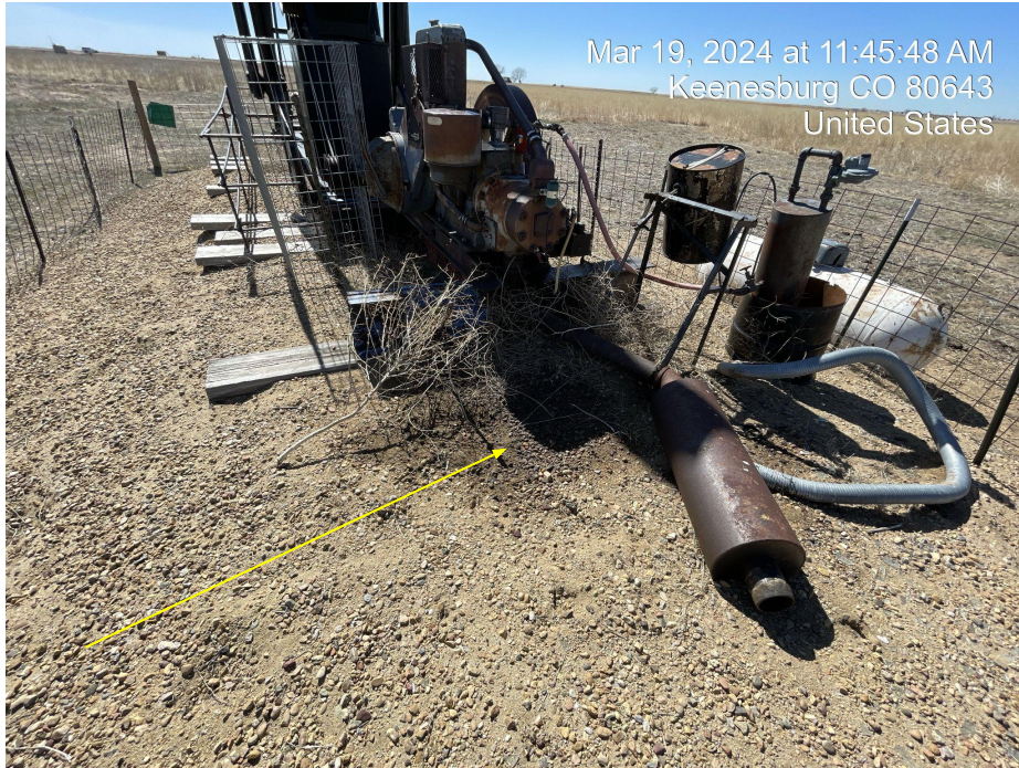
Photo 3. Photo taken facing south of stained soil under pumpjack engine.
