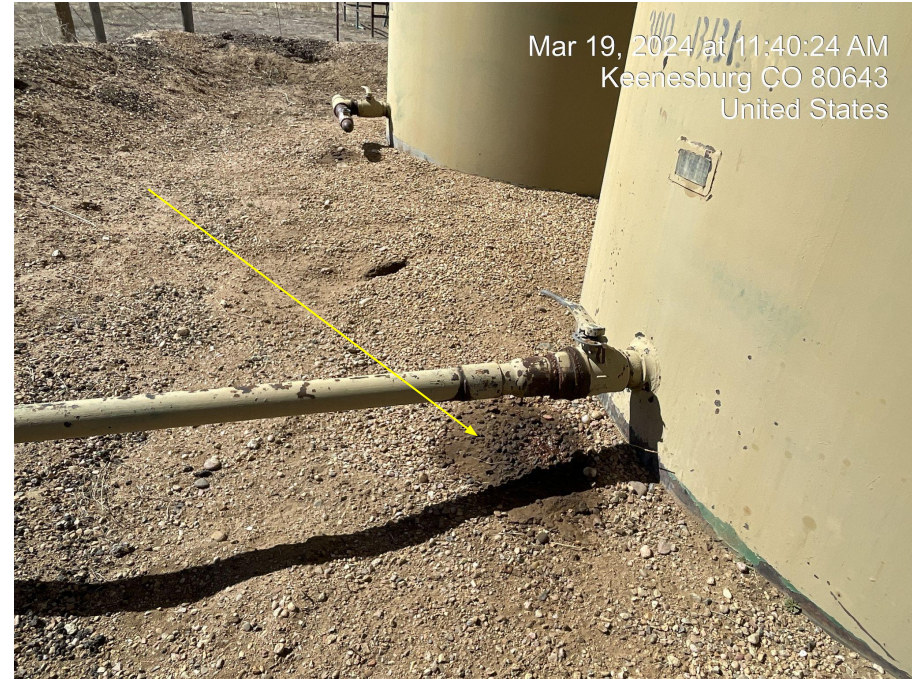
Photo 6. Photo taken facing south of stained soil under tank loadout pipe connection.
