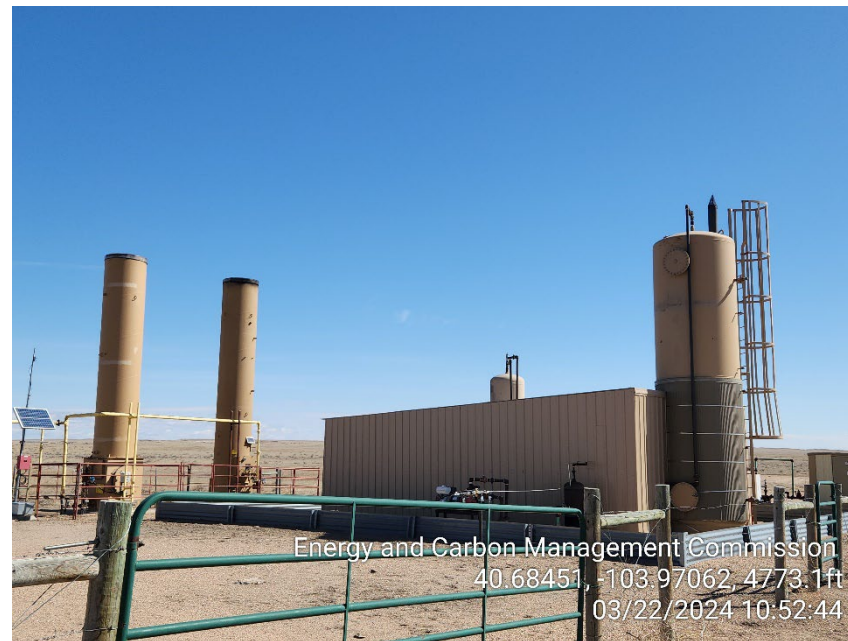
Photo 4 – Heater Treater and ECDs
