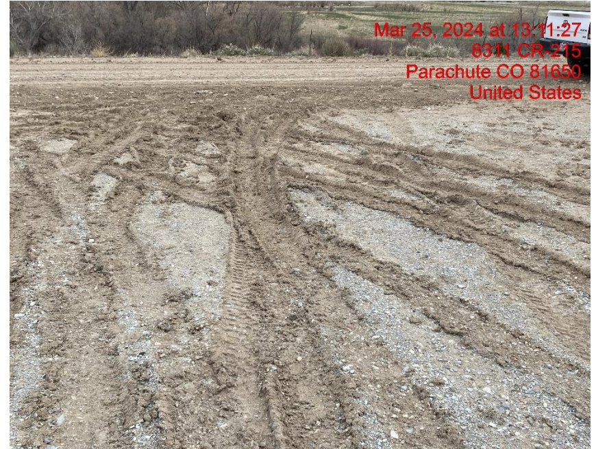
Insufficient Vehicle Tracking BMPs at Location Entrance/Exit – Photo #00035
