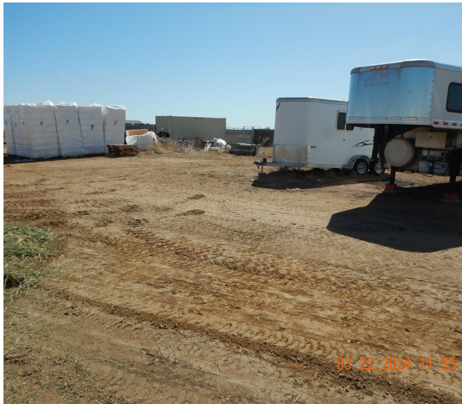
Photo 3. Photo taken from the location, facing South. Photo illustrates all equipment has been removed.
