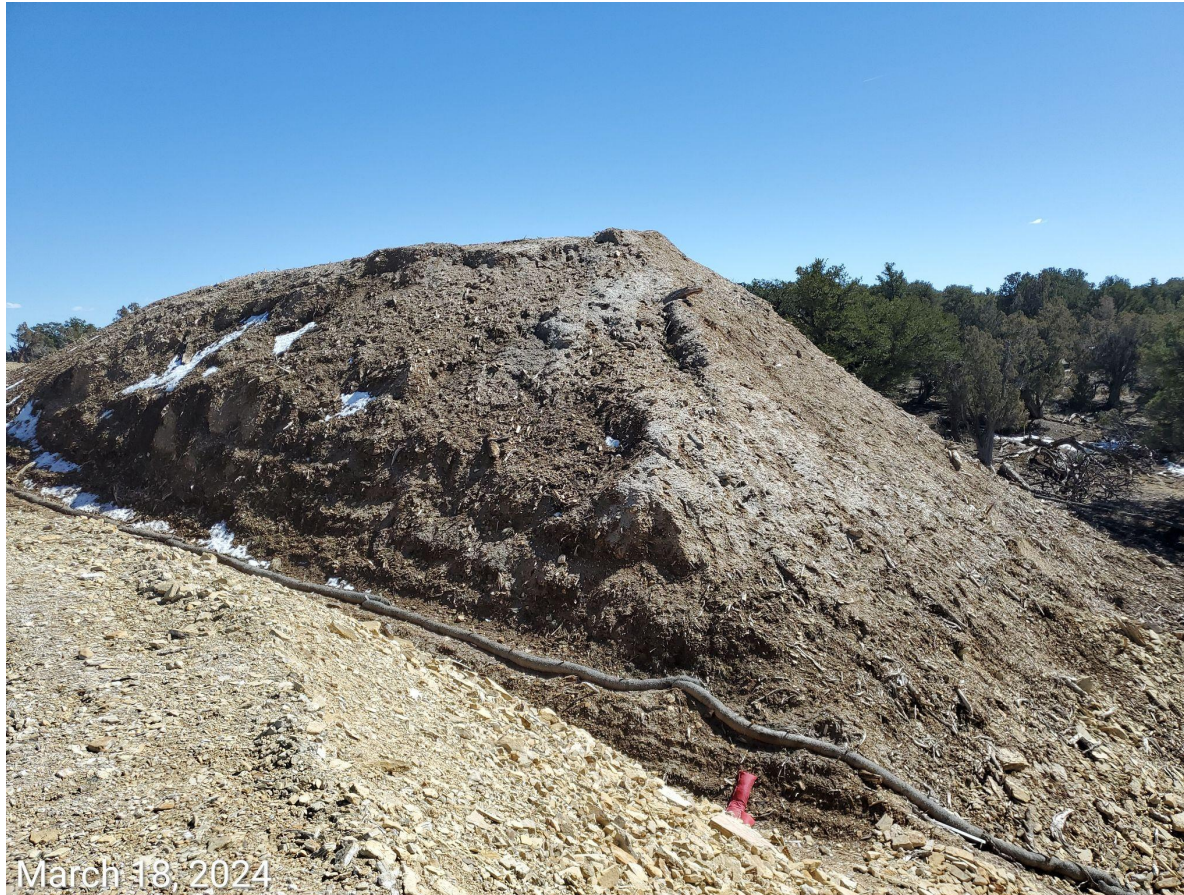
Photo 3: Hydromulch at topsoil stockpile beginning to fail.
