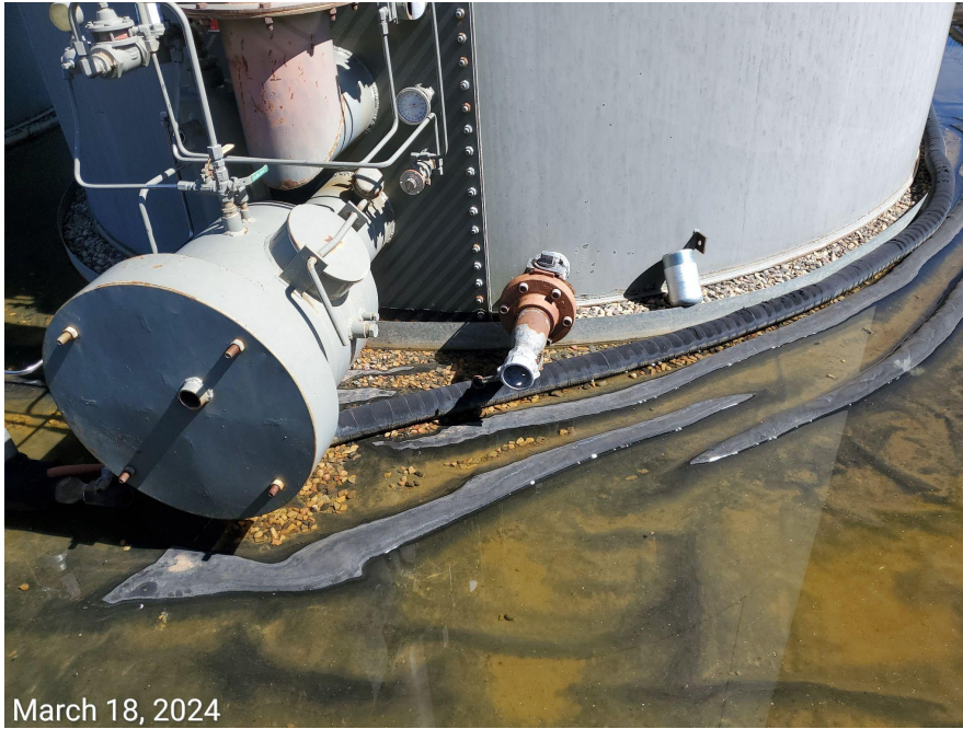
Photo 5: Photos examples showing tanks missing required cap/plug.
