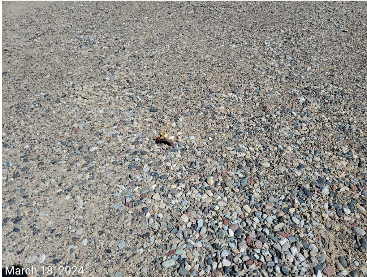
Photo 4: Anchors missing required marking.
