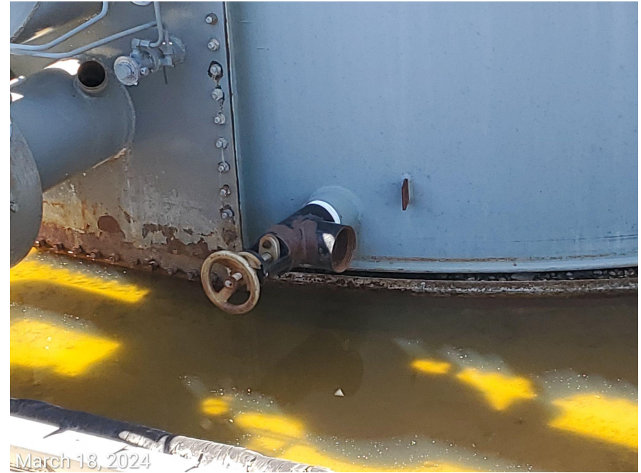
Photo 5: Photos examples showing tanks missing required cap/plug.
