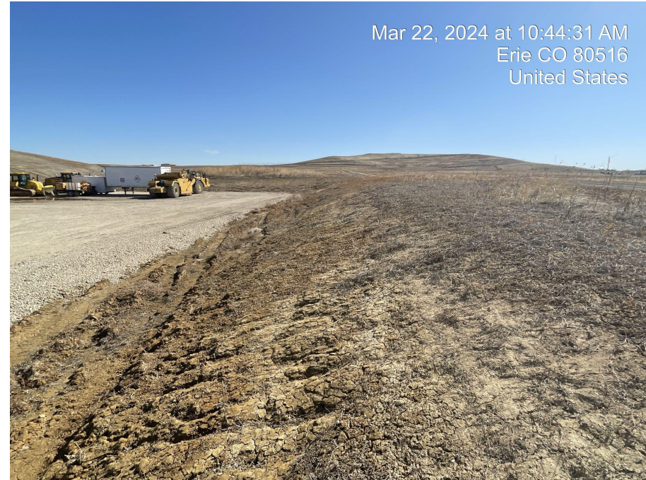
Photo 6. Photo taken facing east of weeds (kochia & russian thistle) and stormwater erosion on south cutslope side of pad.
