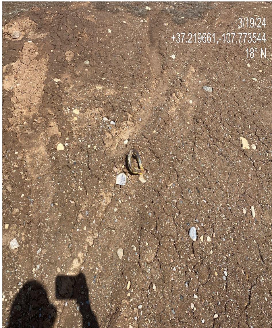
Photo 4. 2 unmarked guy line anchors observed on location.
