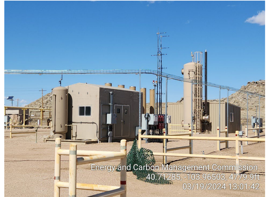
Photo 16 – Instrumental Air Unit and Heater Treater
