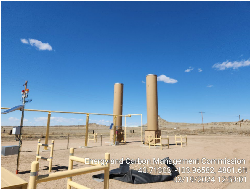
Photo 9 – Produced Water Tanks’ ECDs
