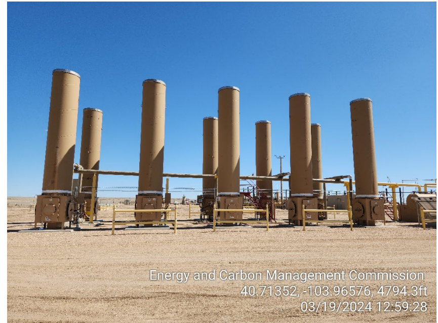
Photo 10 – Crude Oil Tanks’ ECDs
