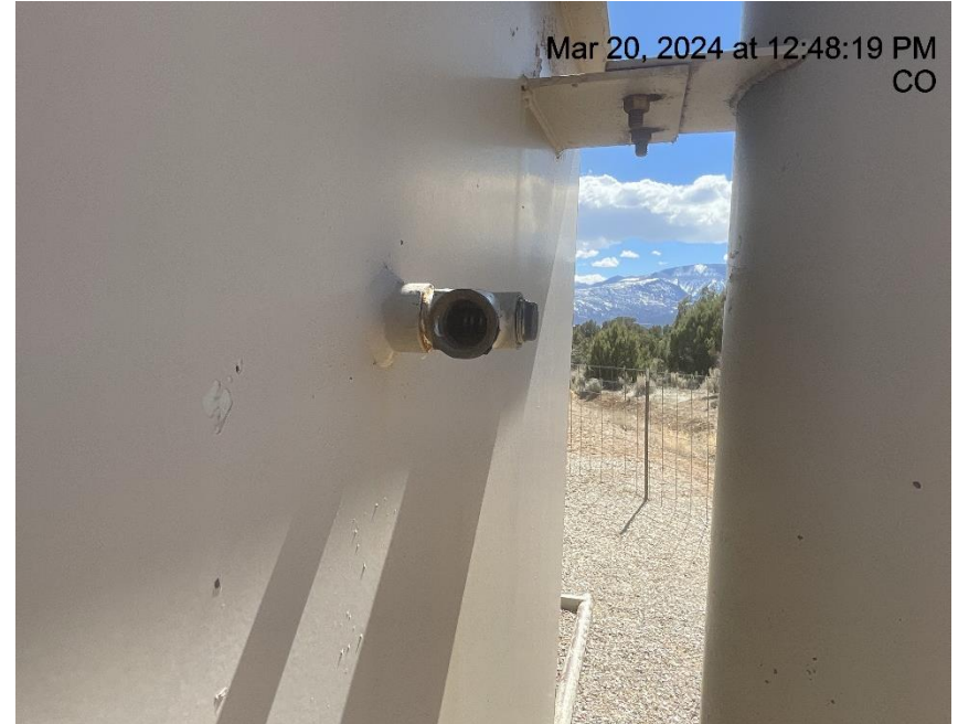
Photo # 675 PRV on separator unit does not comply with CECMC pressure safety device rules & general safety rules.
