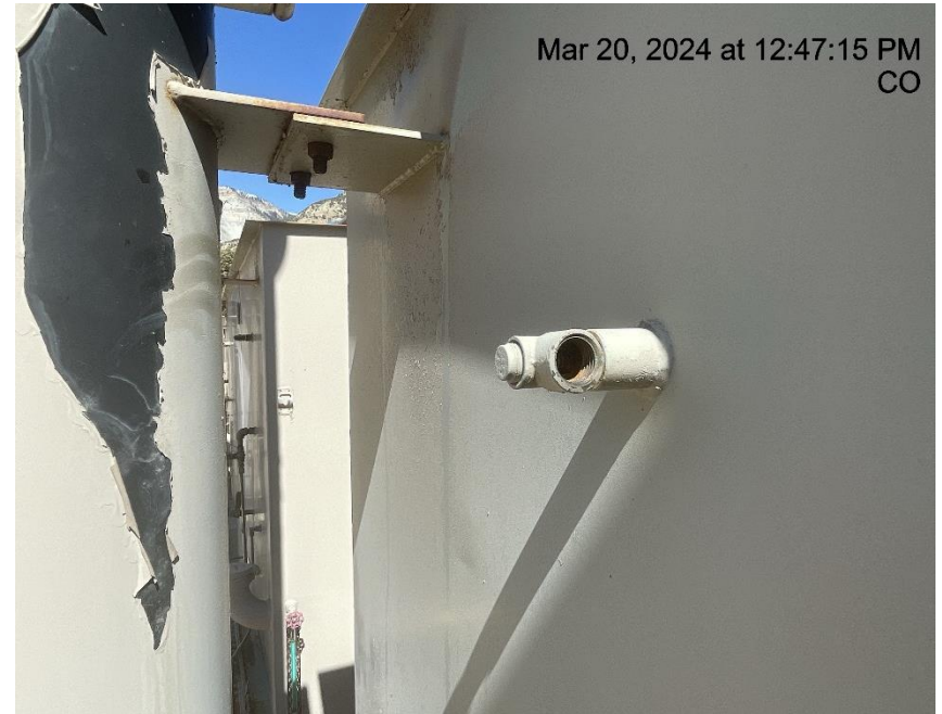
Photo # 671 PRV on separator unit does not comply with CECMC pressure safety device rules & general safety rules.
