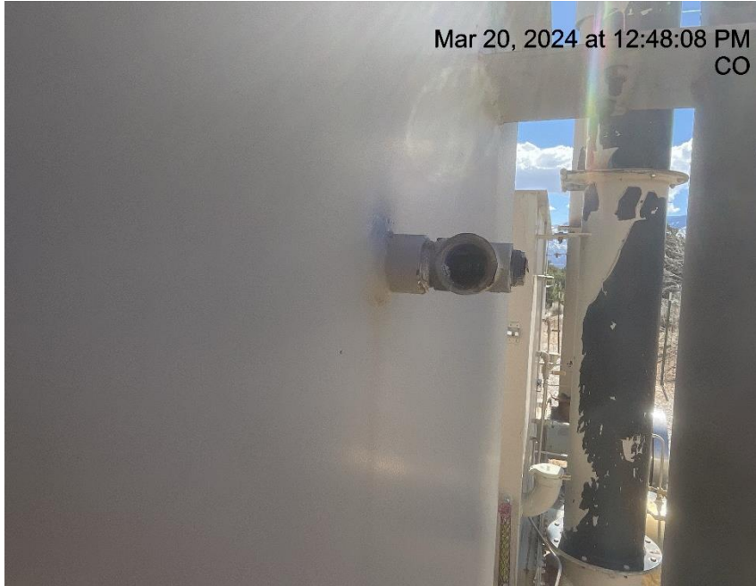
Photo # 674 PRV on separator unit does not comply with CECMC pressure safety device rules & general safety rules.
