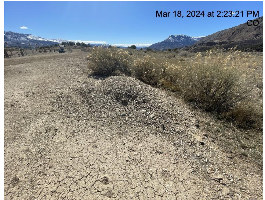
Photo # 326 Stockpiled soils with no BMP's
