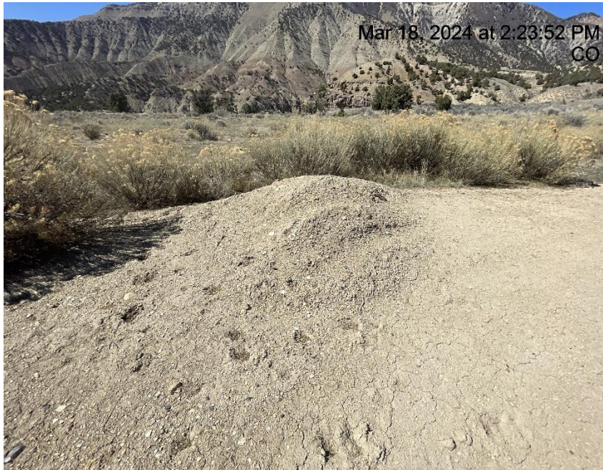
Photo # 325 Stockpiled soils with no BMP's
