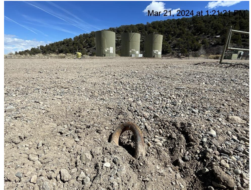
Photo # 1041 Same unmarked deadman from a different angle
