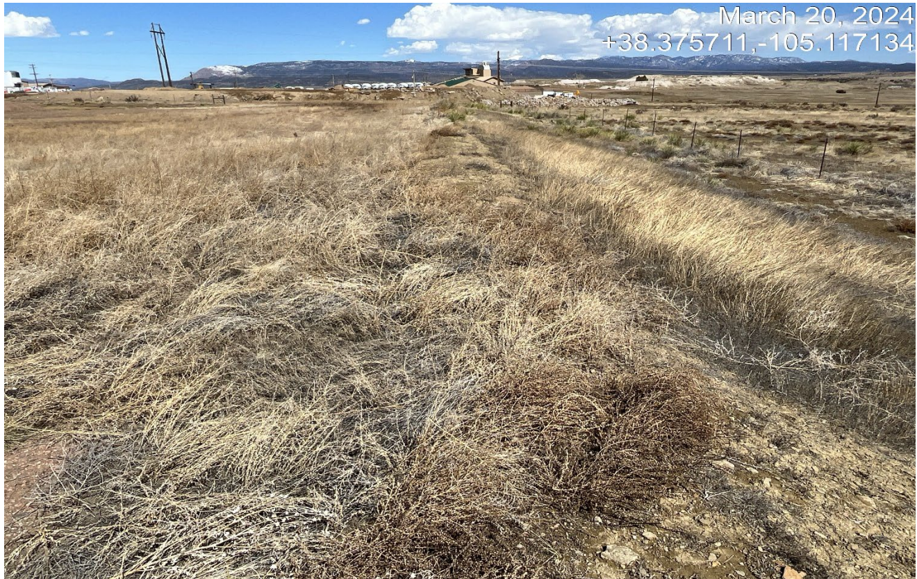
Photo 5. Southeast corner of the location facing north along the fill slope. There are undesirable growing along the fill slope that need to be controlled. The location has not been recontoured. Previous corrective action was not completed.
