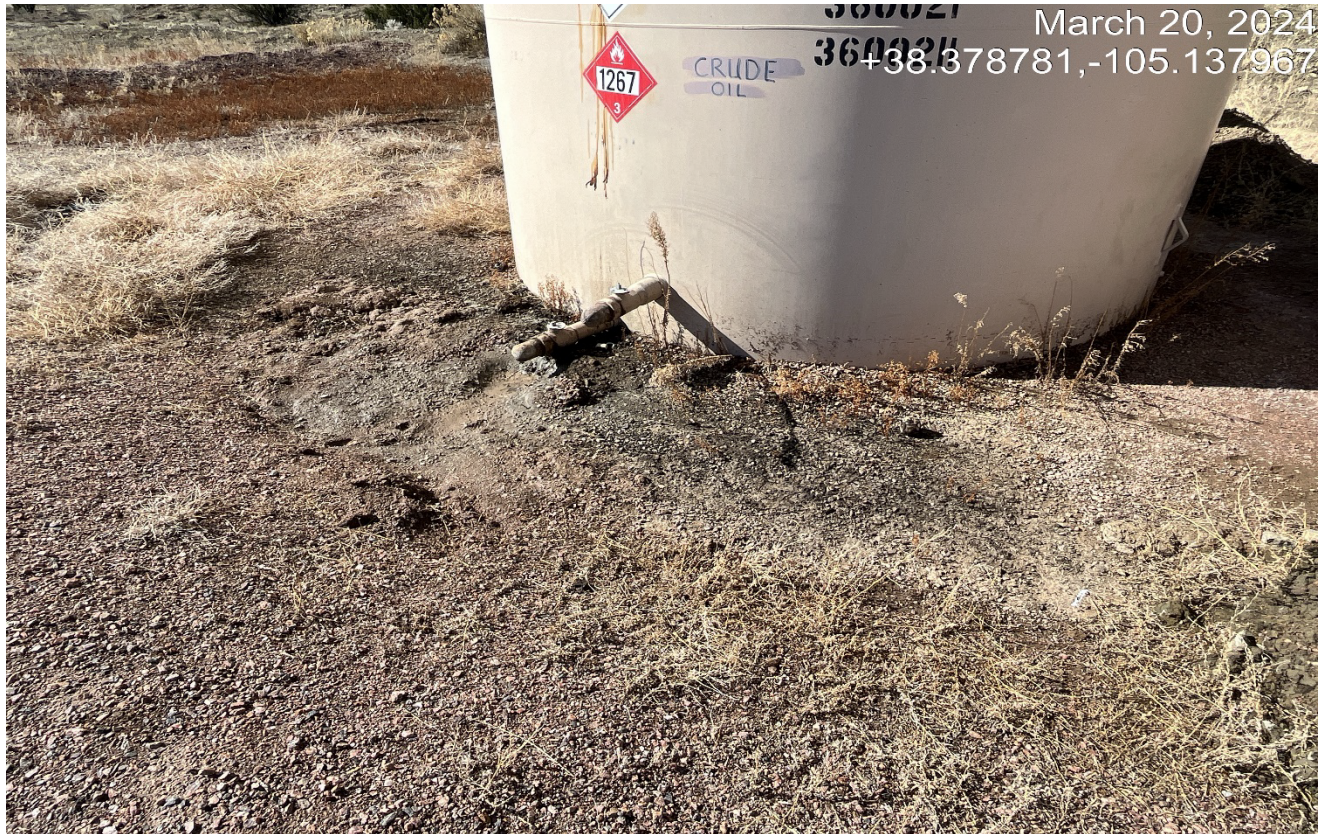
Photo 6. Upon closer inspection of the tanks there is a spill that had occurred at the tank outlet. Immediate clean up needs to be performed.
