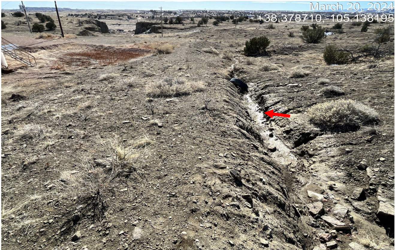
Photo 8. Facing southeast at the south side of the location. There is an erosion channel shown at red arrow which will need to be repaired and stabilized.
