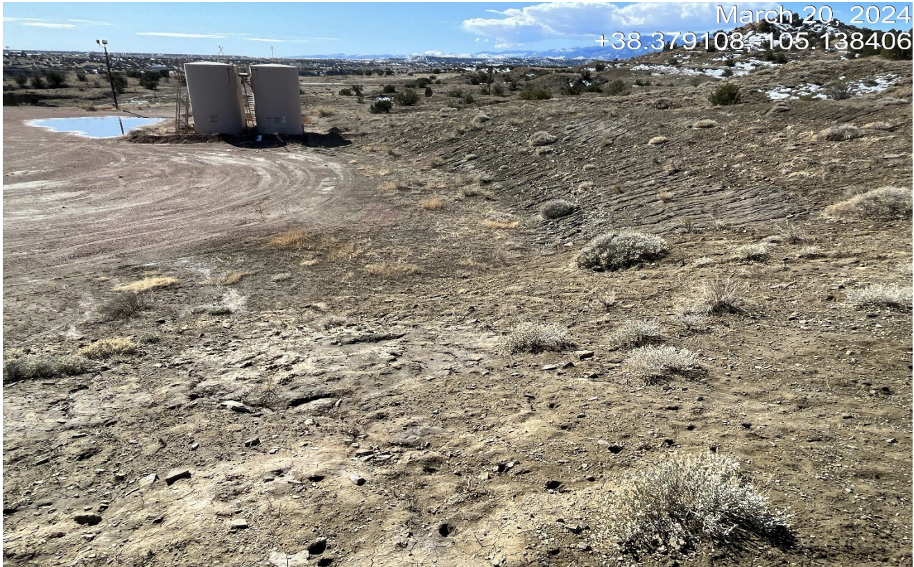
Photo 9. Facing east along the cut slope. There are rilling erosion along the cut slope.
