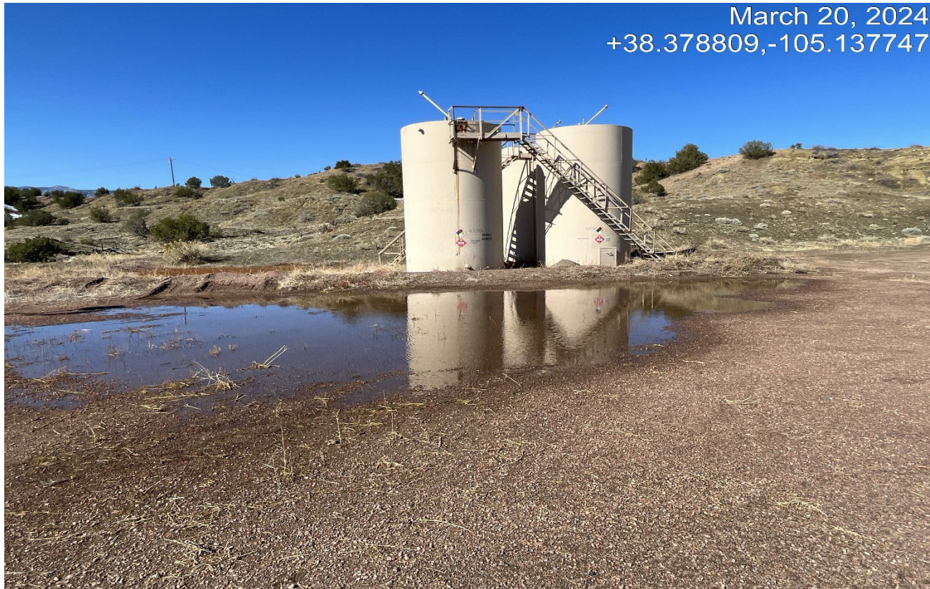
Photo 5. Facing toward the south side of the location. There are tanks that have not been removed. All equipment should have been removed within 3 months of abandonment.
