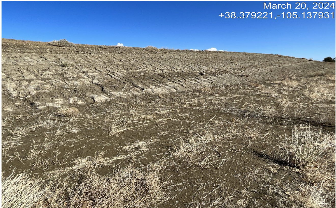
Photo 10. Facing northwest along the cut slope. There cut slope is not stabilized.
