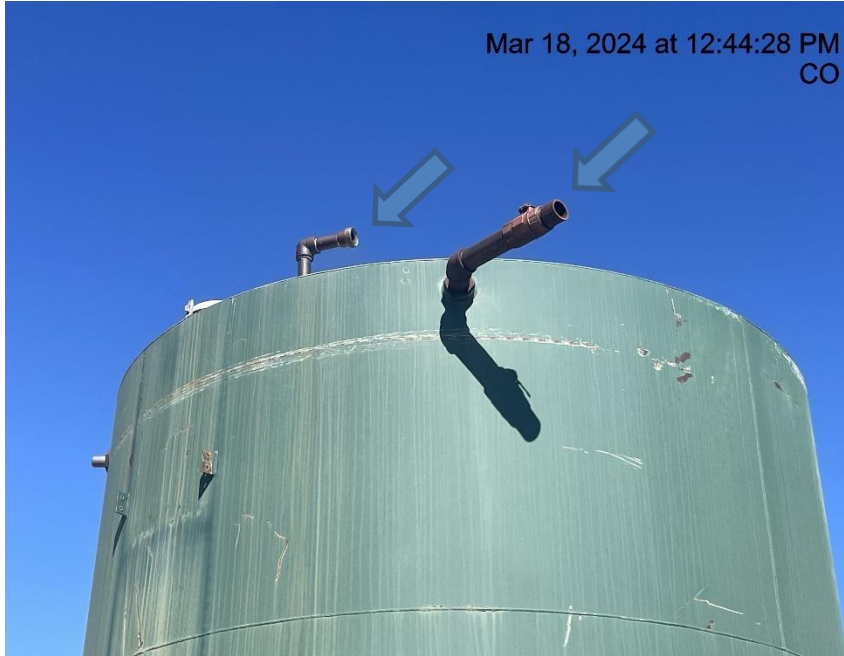
Photo # 230 Open ended piping on unused equipment is a wildlife hazard
