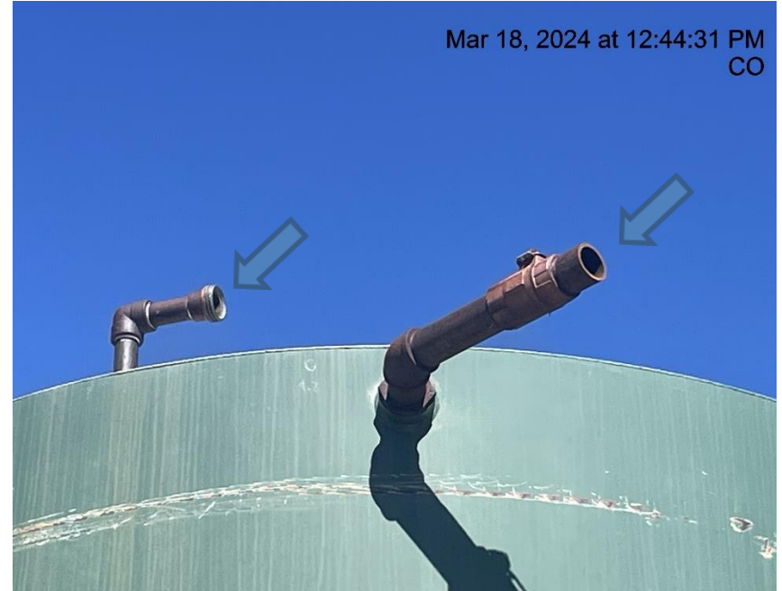
Photo # 232 Open ended piping on unused equipment is a wildlife hazard
