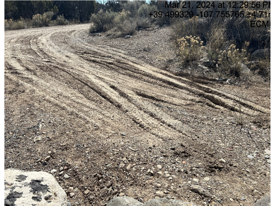
Lack of stabilization/compaction
