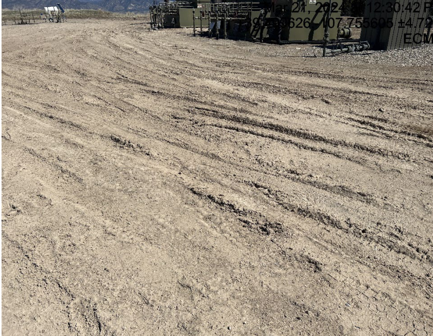
Lack of stabilization/compaction
