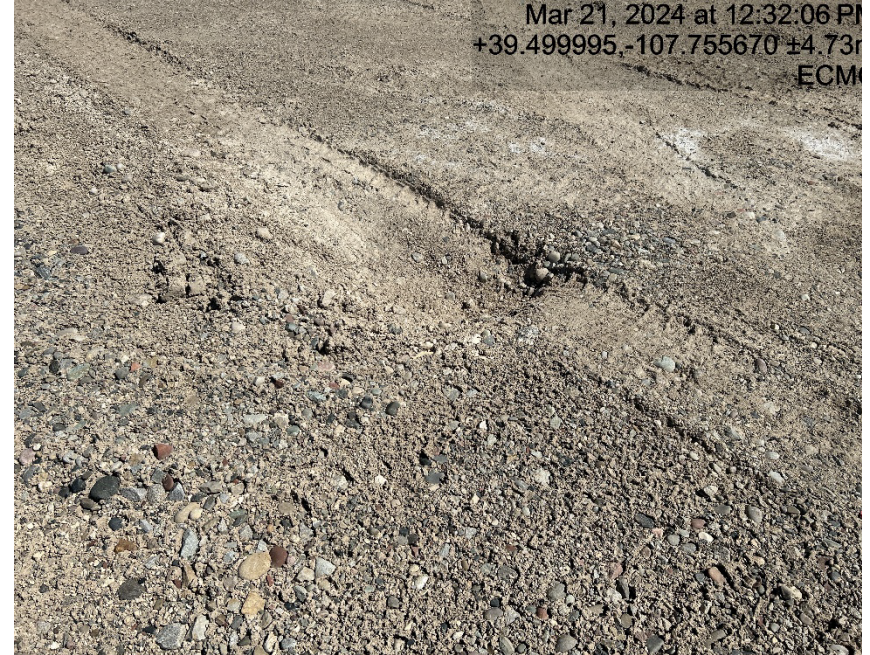
Lack of stabilization/compaction
