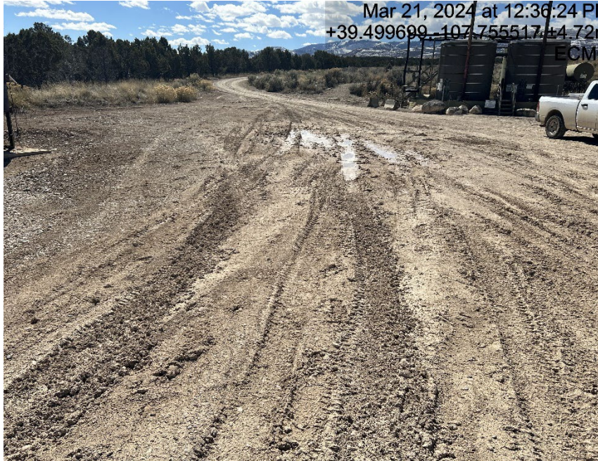
Lack of stabilization/compaction
