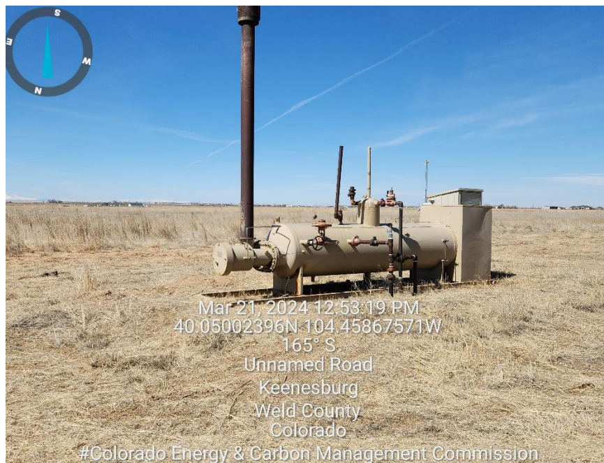
Photo 3 Heater stack installed Dead vegetation around separator
