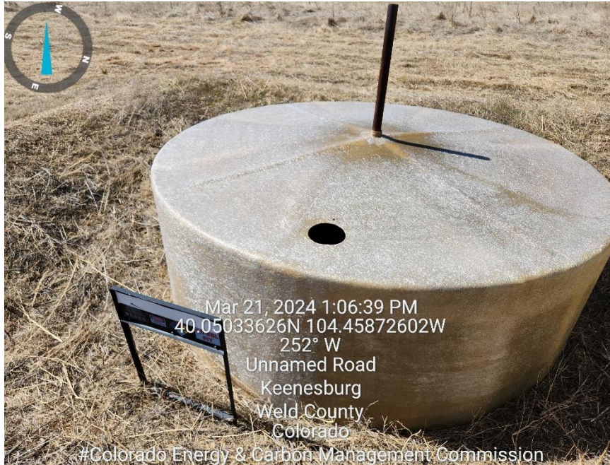
Photo 9 Wildlife protection hole in produced water tank
