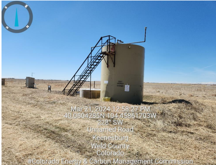
Photo 7 Oil tank has no placards or volume signs
