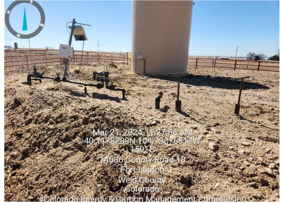
Photo 4 risers not ooslat tagged. Meter no card and meter is non operational
