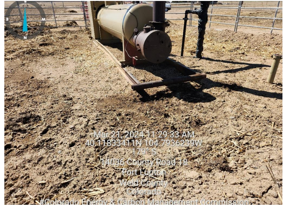
Photo 10 Mechanical issue and stained soil on ground of Hoz sep.
