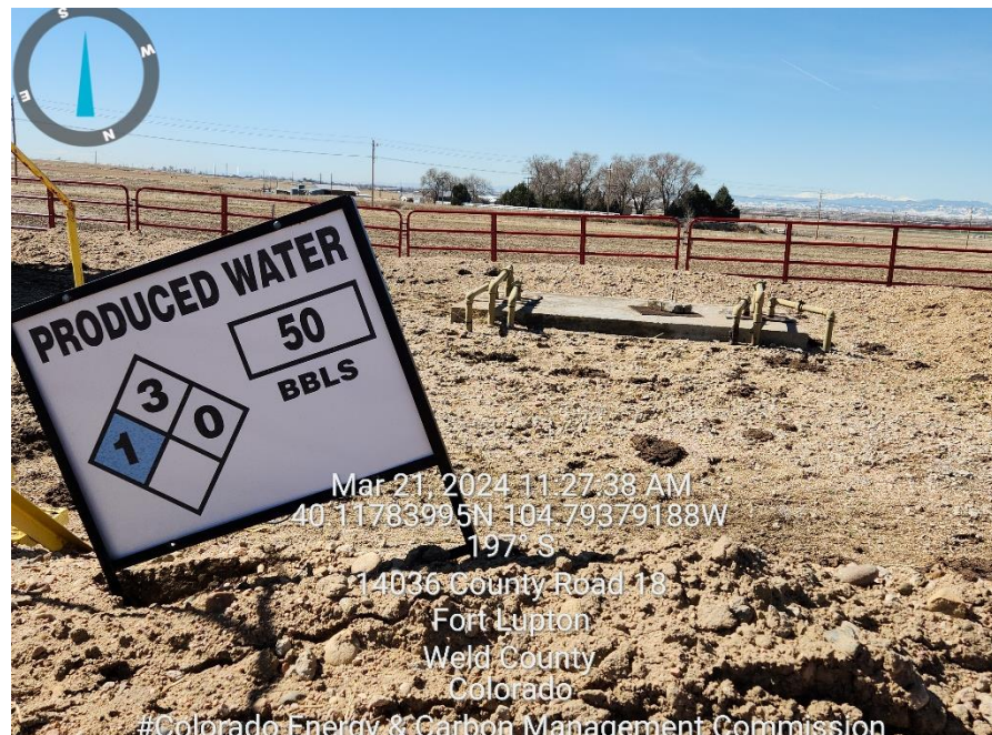
Photo 6 Produced water vault NFPA Placard faded.
