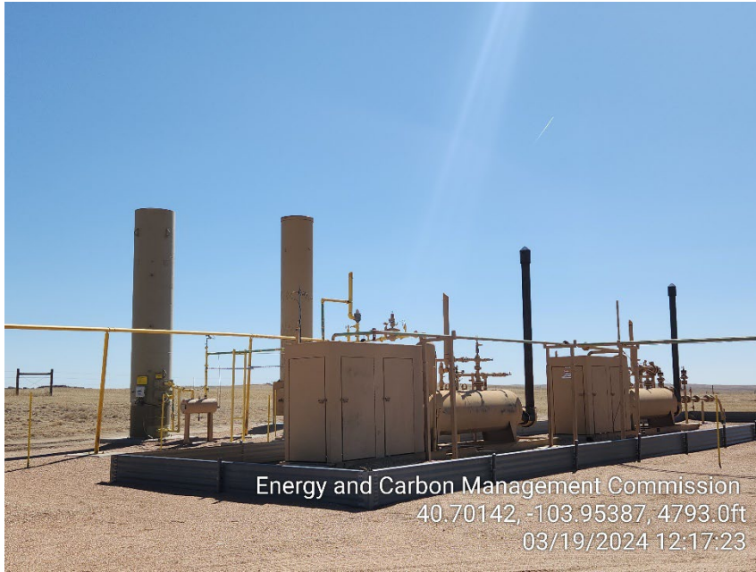
Photo 3 – Separators and ECDs
