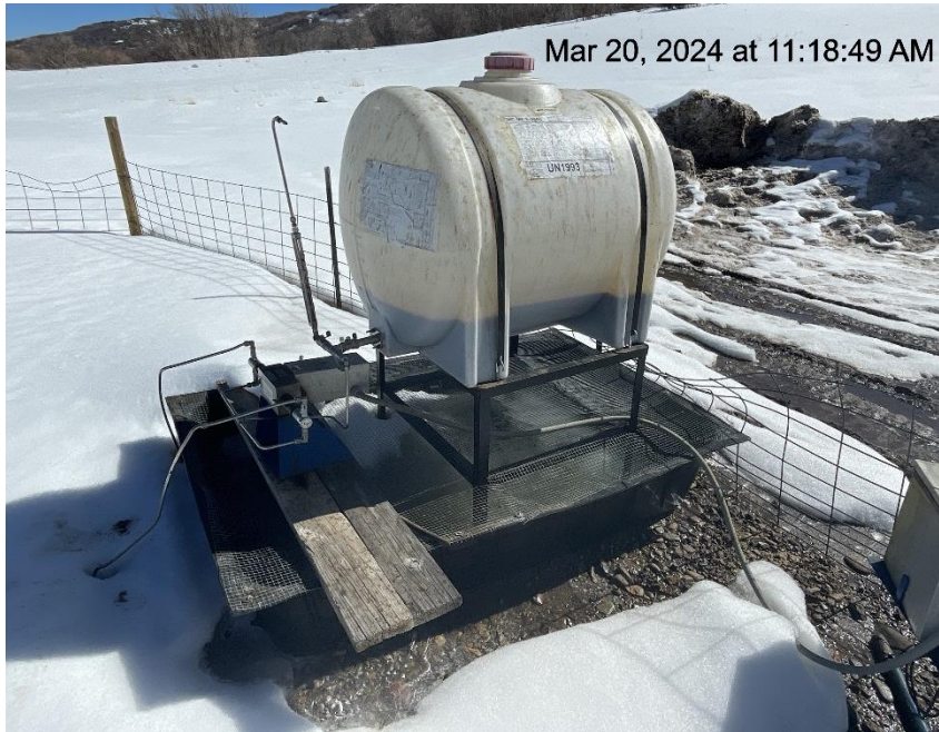
Photo # 617 Chemical tank containment approximately 5/8 to 3/4 full of fluid/Failure to maintain chemical BMP
