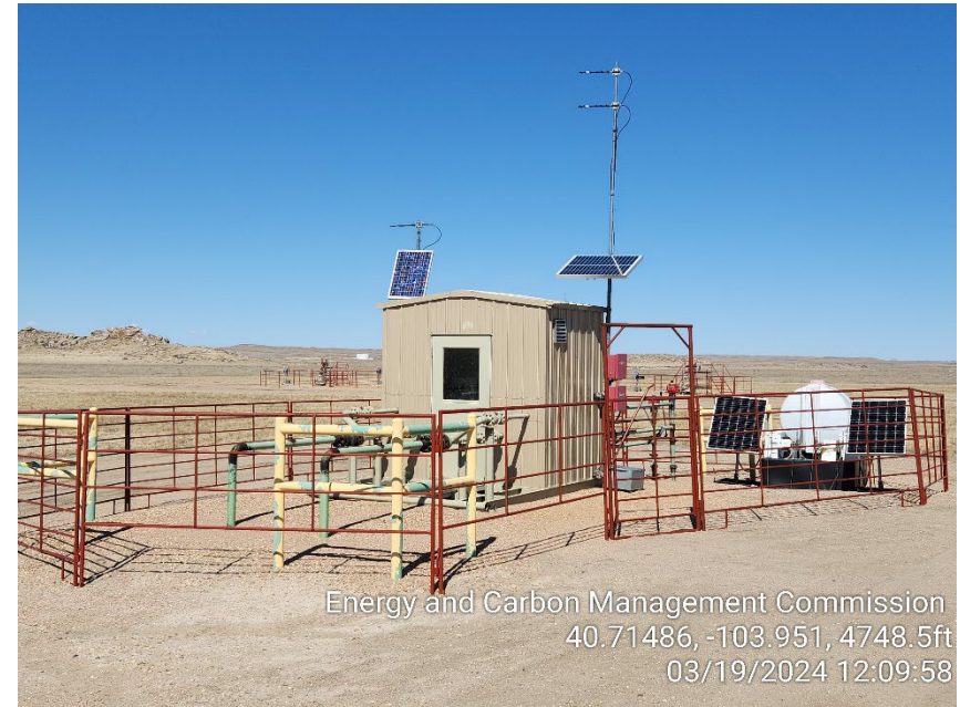
Photo 6 – Gas Lift Injection Meter House
