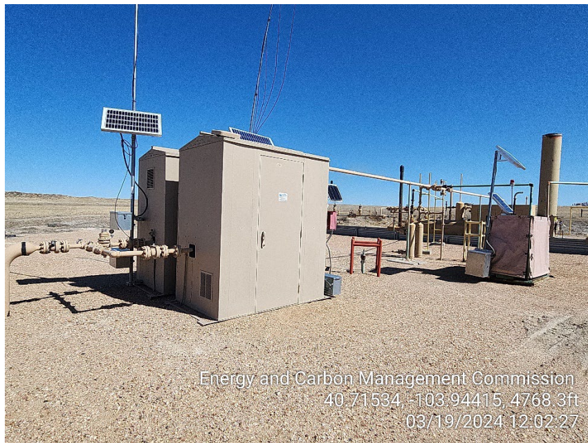
Photo 9 – Gas Meters and VRU
