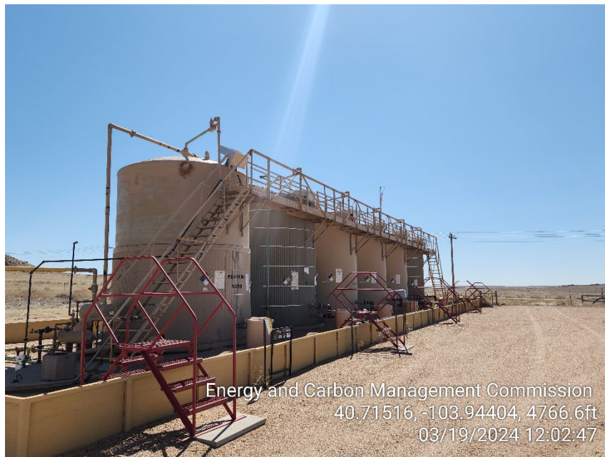
Photo 11 – Tank Battery
