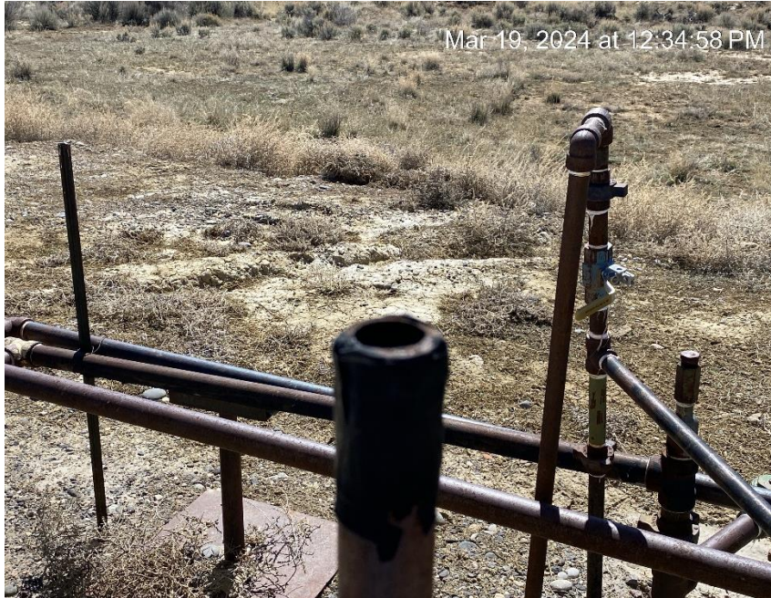
Pop off riser missing rain protection
