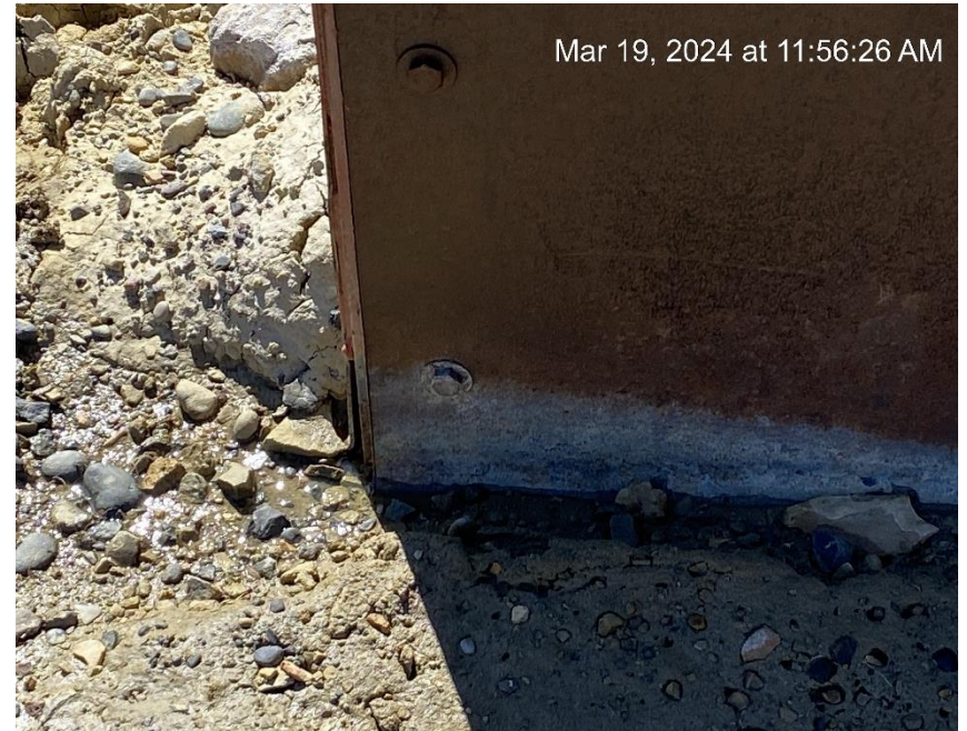
Leaking containment
