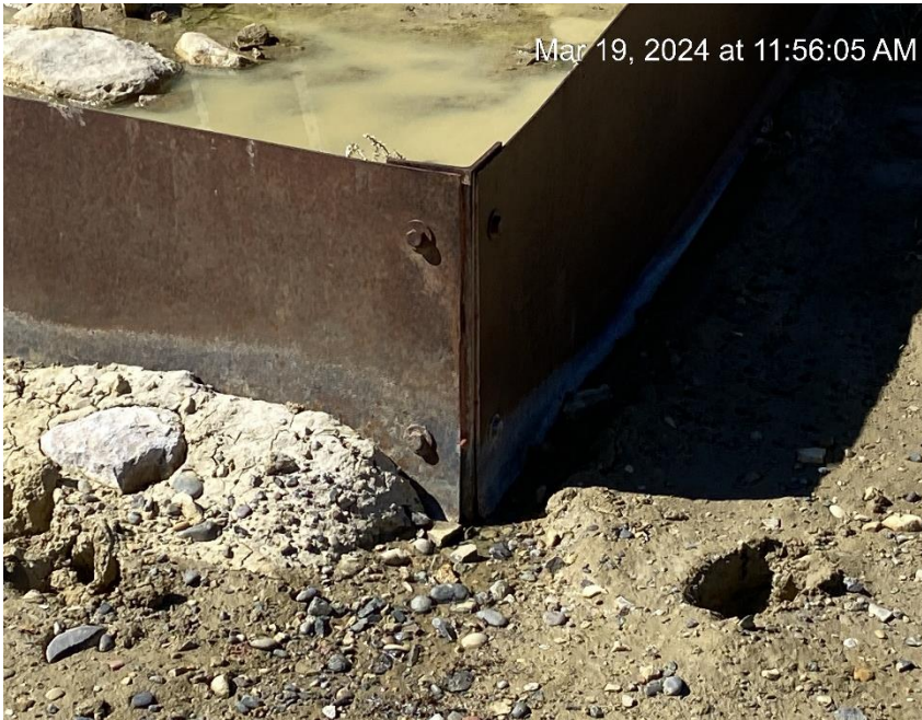
Containment leak
