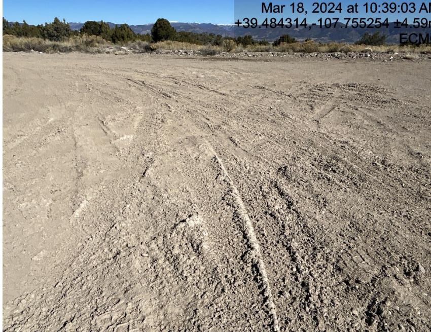
Lack of stabilization/compaction
