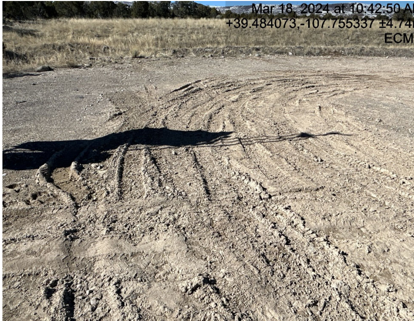
Lack of stabilization/compaction
