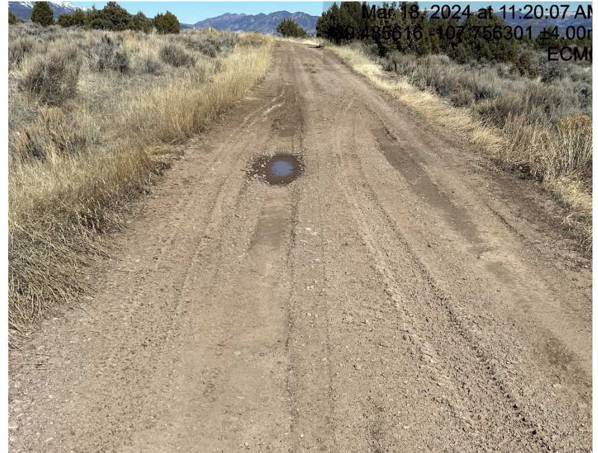
Lack of stabilization/compaction
