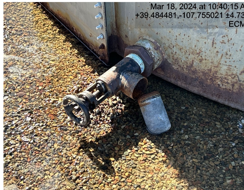
Cap not installed properly
