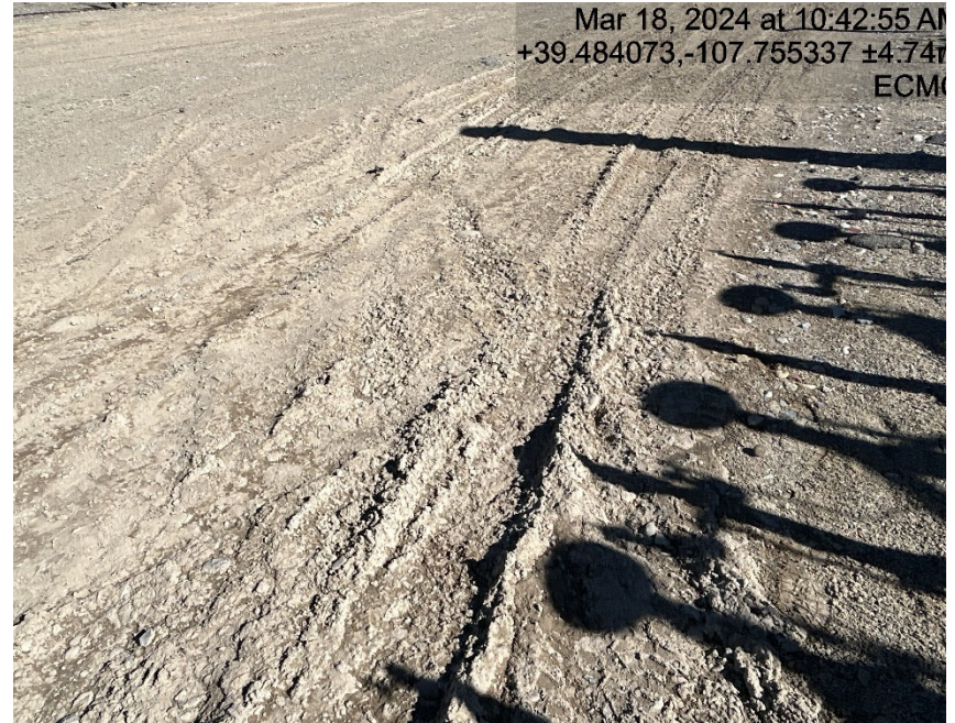
Lack of stabilization/compaction
