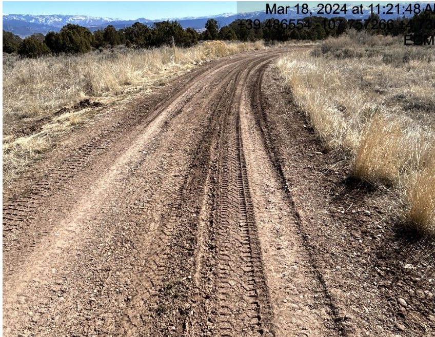
Lack of stabilization/compaction
