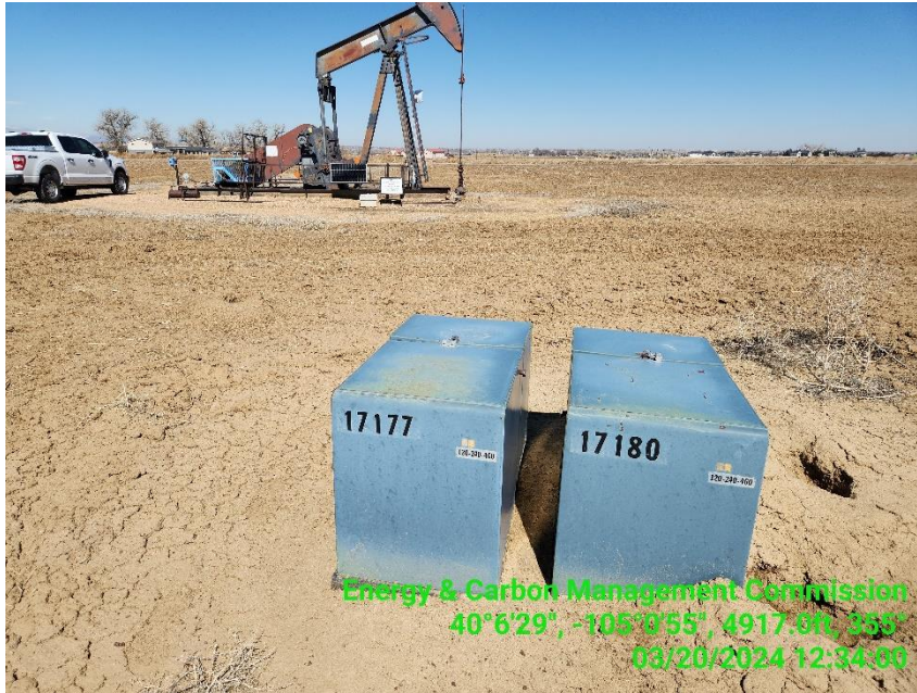
Photo 9 Unused transformers facing the wellsite.
