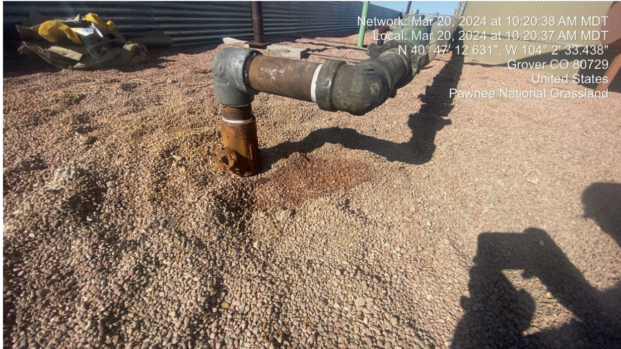
Photo Date 3/20/2024- Impacted soil from release.
