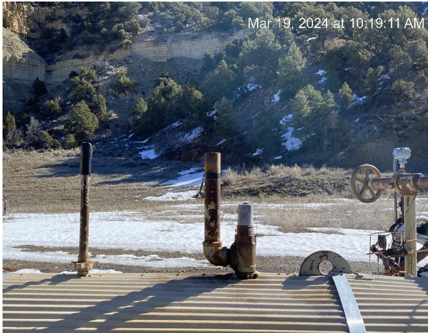
Relief riser missing rain protection
