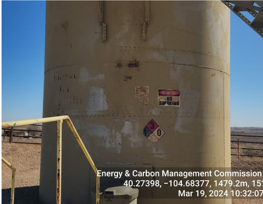
Photo 9: No contents/capacity displayed
