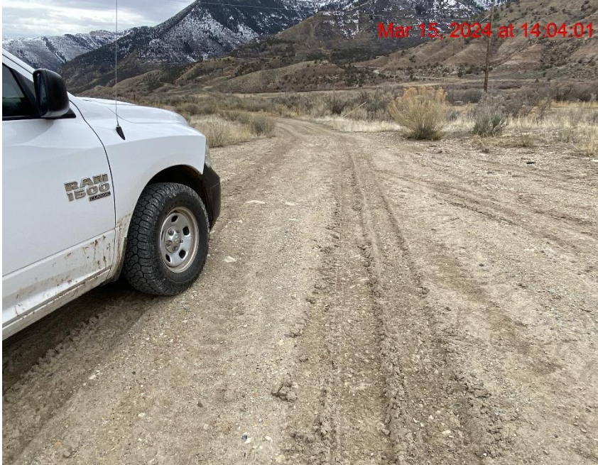
Insufficient Vehicle Tracking BMPs at Location Entrance/Exit – Photo #00002
