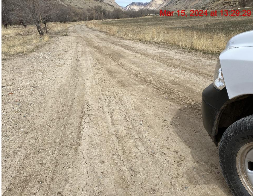
Insufficient Vehicle Tracking BMPs at Location Entrance/Exit – Photo #09962
