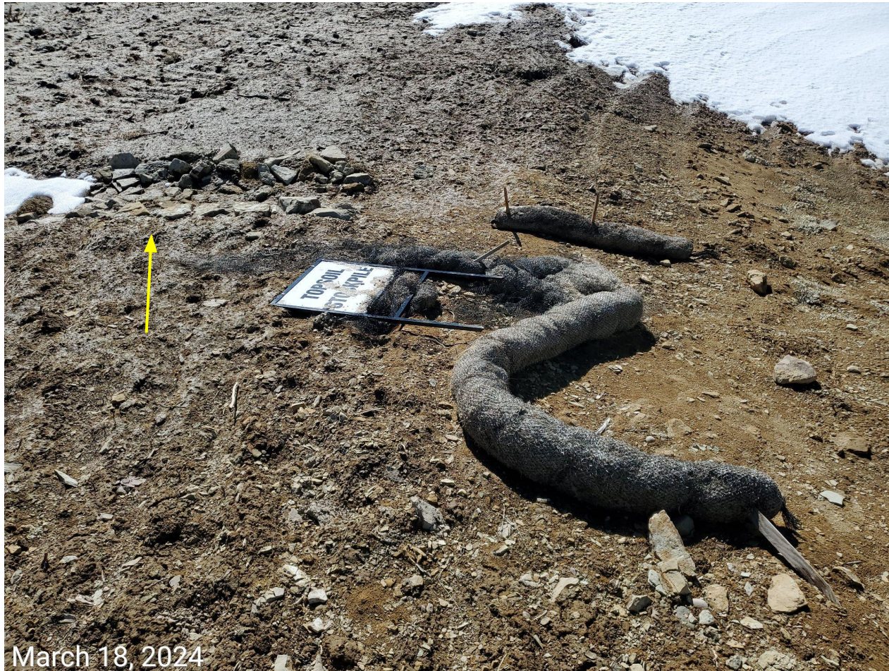
Photo 4: Photo taken from the sediment trap on the south end of the Location. Photo shows unused signage and wattles; this is now considered debris. Photo also shows inlet to trap appears inadequate in size.
