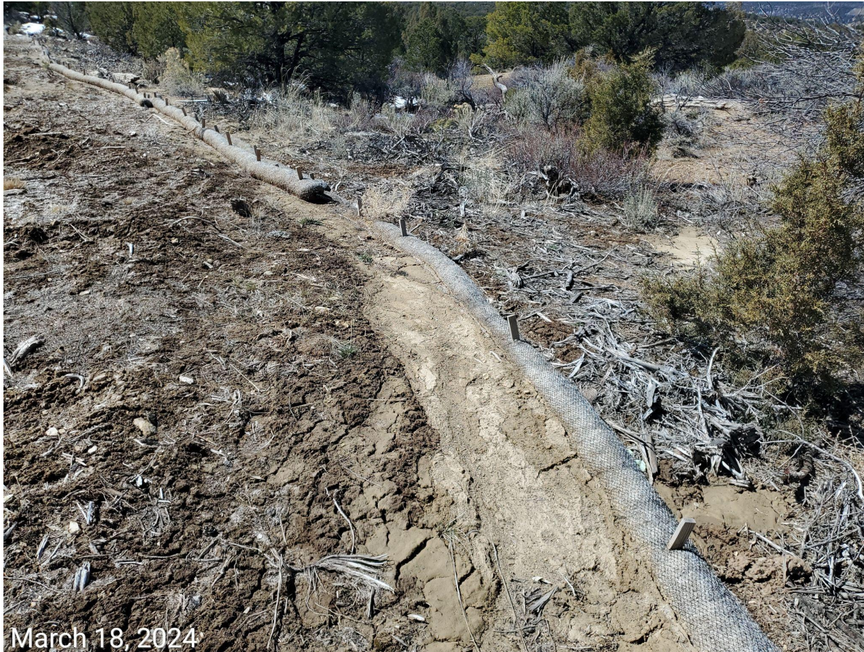
Photo 5: Photo example showing erosion logs along perimeter of the Location have filled with sediment.
