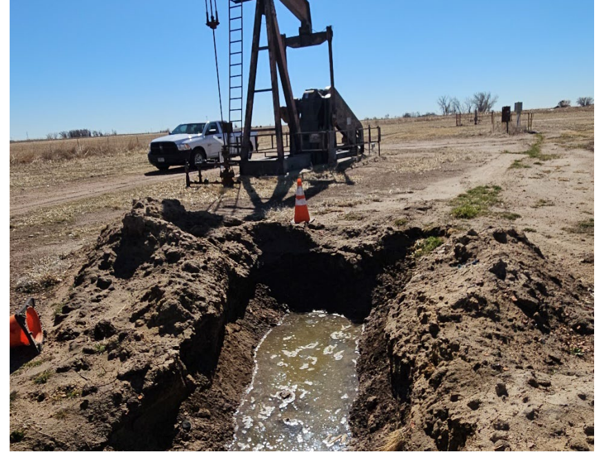
Open excavation without fencing or storm water BMPs
