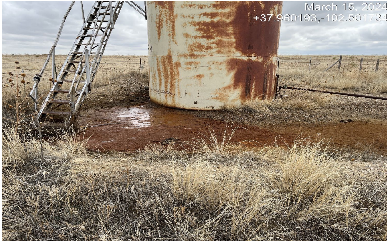
Photo 3. Facing east toward the tank. There is a leak that occurred at the tank within the secondary containment. There is insufficient labeling and signage at the tank .
