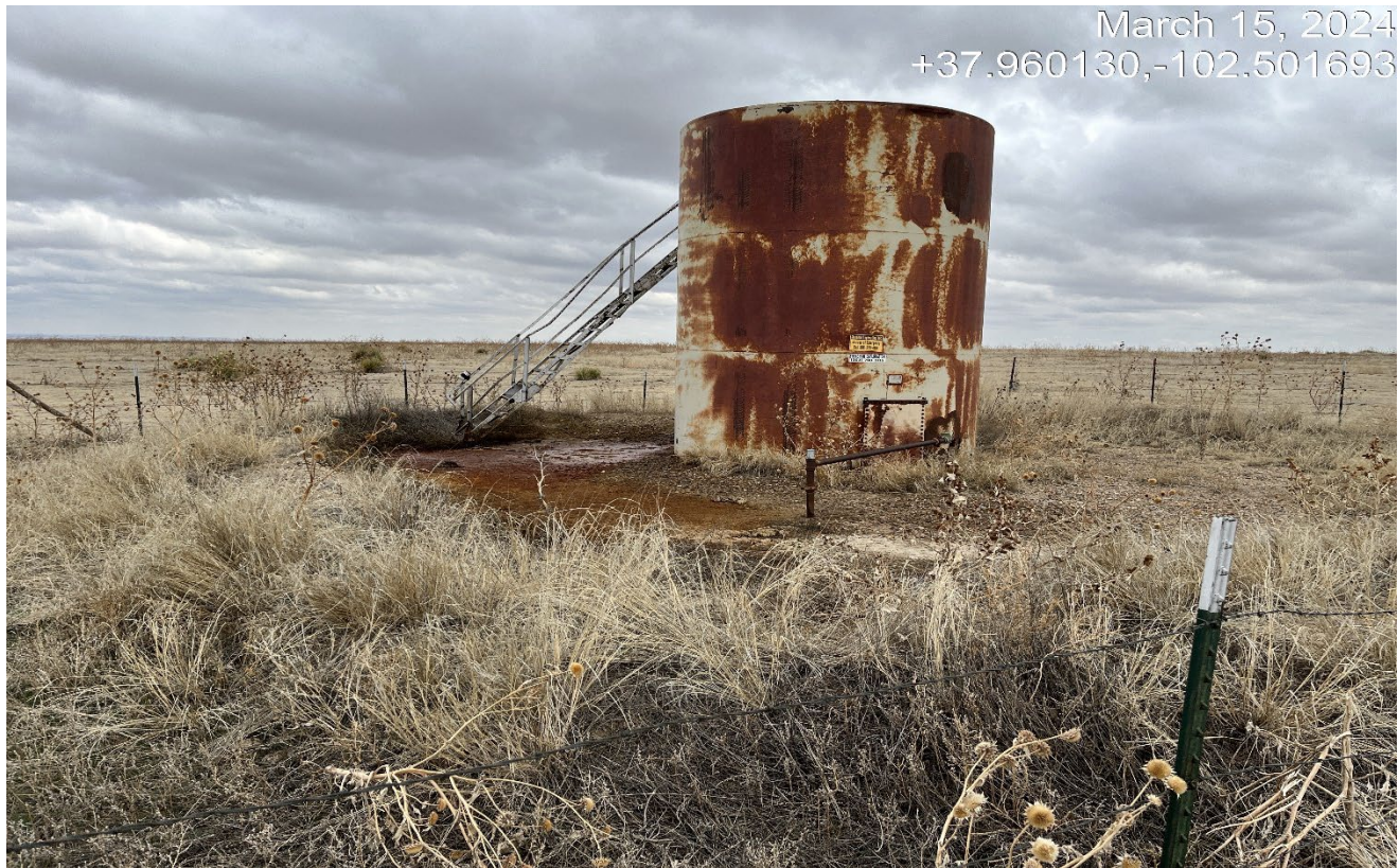
Photo 2. Facing northeast toward the tank. There is a leak that occurred at the tank within the secondary containment. There is insufficient labeling and signage at the tank .
