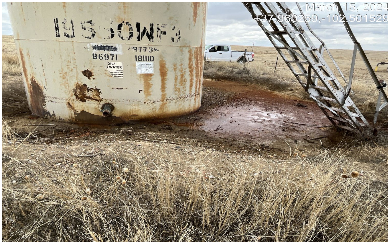
Photo 4. Facing toward the tank. There is a leak that occurred at the tank within the secondary containment. There is insufficient labeling and signage at the tank .
