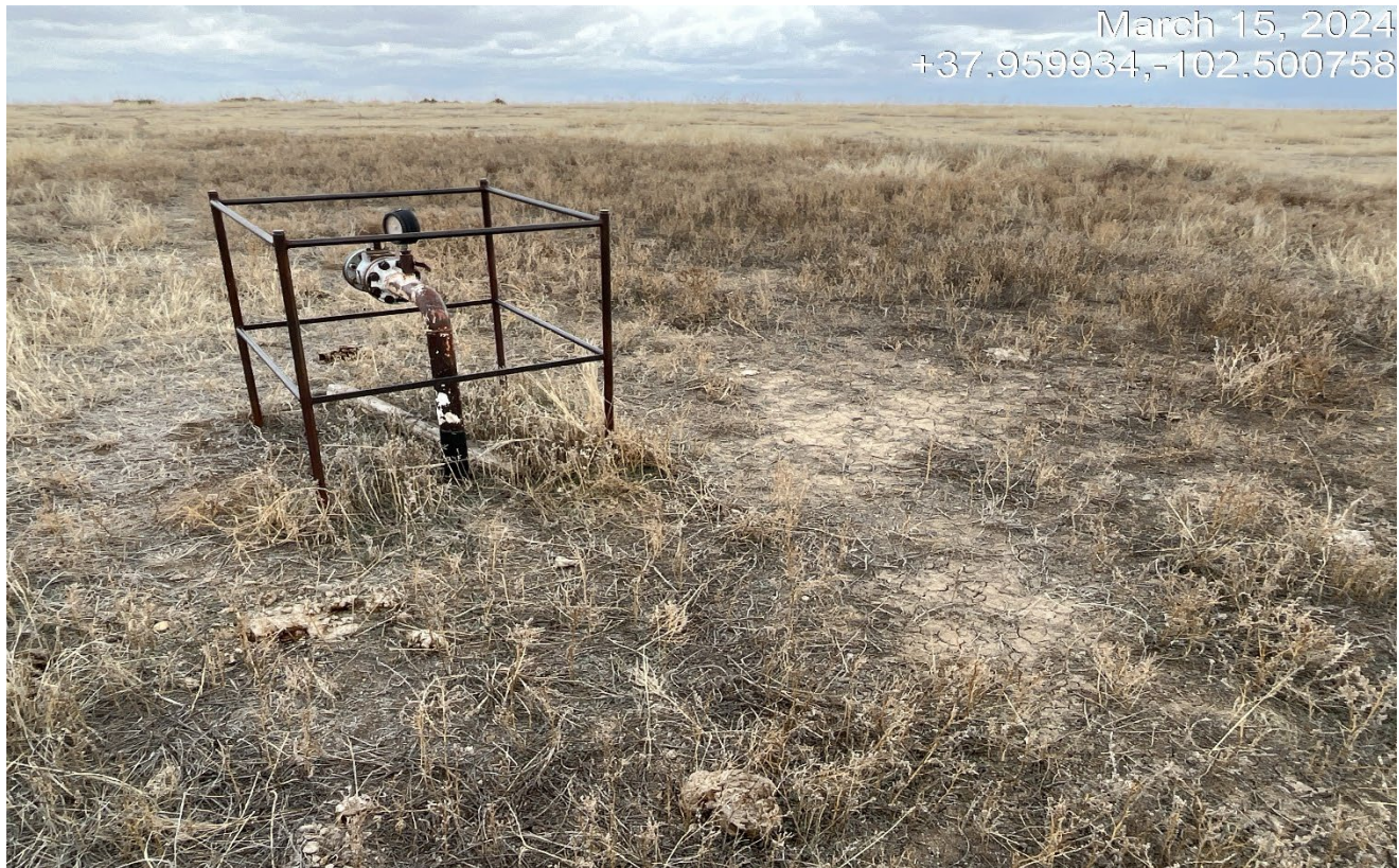
Photo 2. There is an abandoned pipe riser that remains on location that was never removed..
