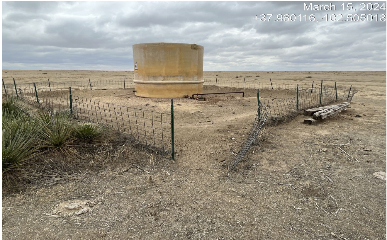
Photo 3. Facing toward the fiberglass tank. The fence around the tank is not maintained to prevent livestock entry.
