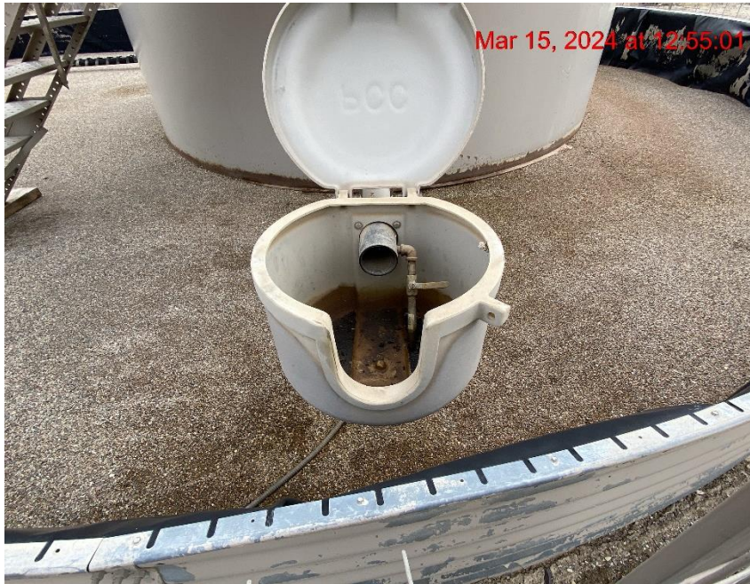
Open-Ended Load Line – Photo #09925
