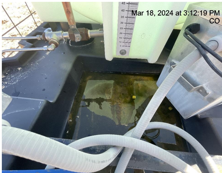
Photo # 388 Chemical containment approximately \frac{3}{4} full of fluid/Failure to maintain chemical BMP/BMP insufficient to contain possible spill.
