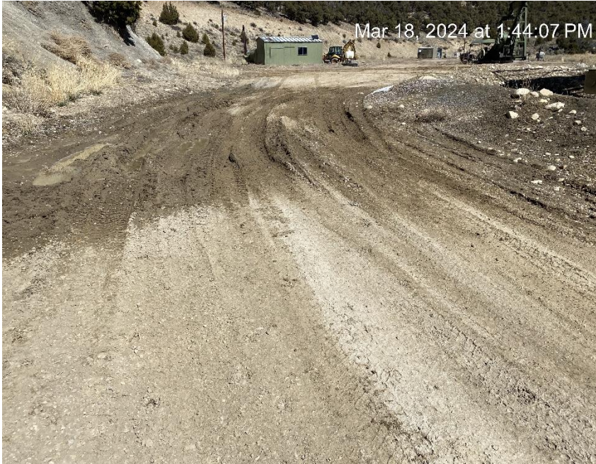
Lack of Stormwater BMP maintenance and vehicle tracking
