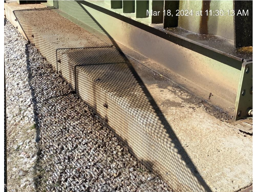
Oily waste and soil staining
