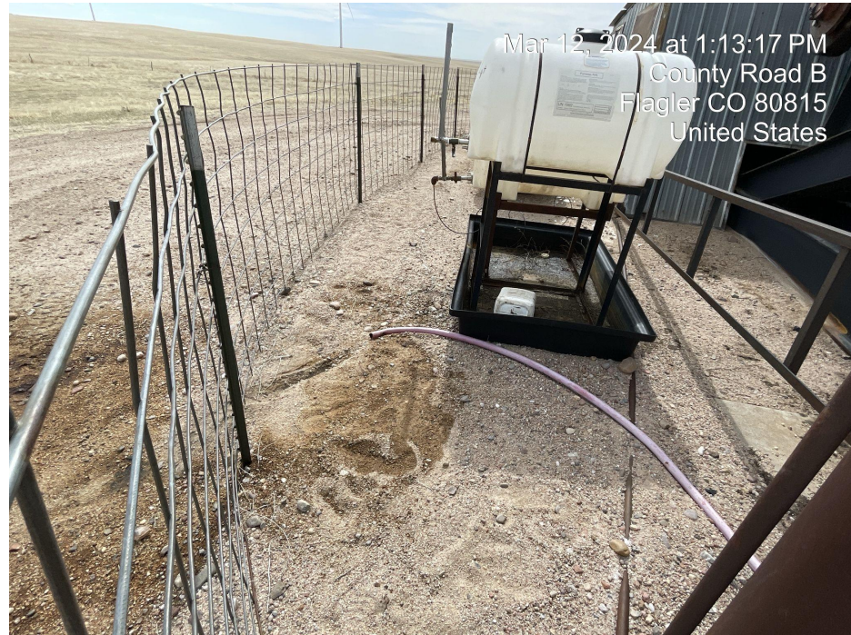
Photo 4. Photo taken facing east of secondary containment without wildlife protection, and stained soil from spill onsite.
