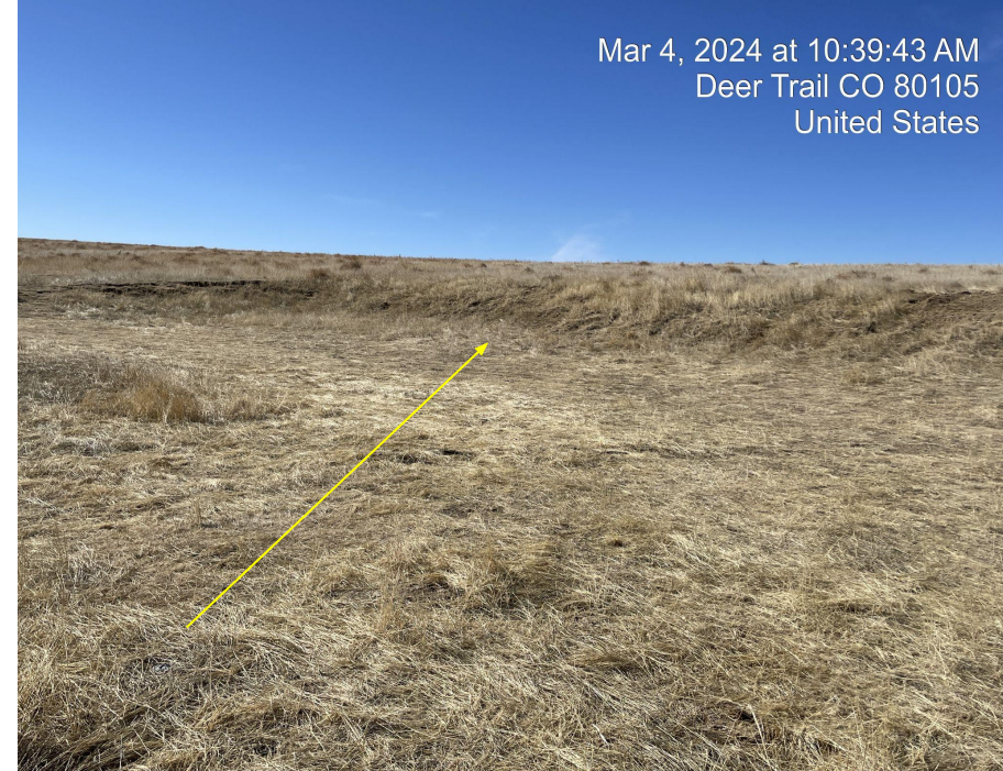
Photo 6. Photo taken facing southwest of vegetation and cut slope that has not been recontoured in reclamation area. Yellow arrow indicates cut slope.
