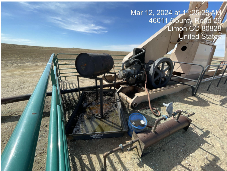
Photo 3. Photo taken facing northeast of secondary containment lacking wildlife protection.
