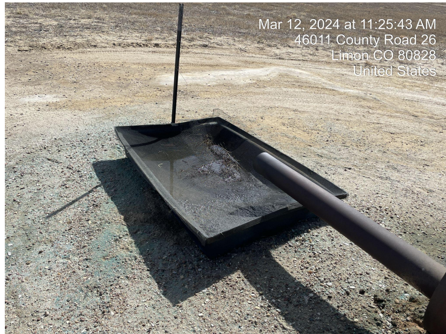
Photo 4. Photo taken facing northeast of secondary containment with wildlife protection.
