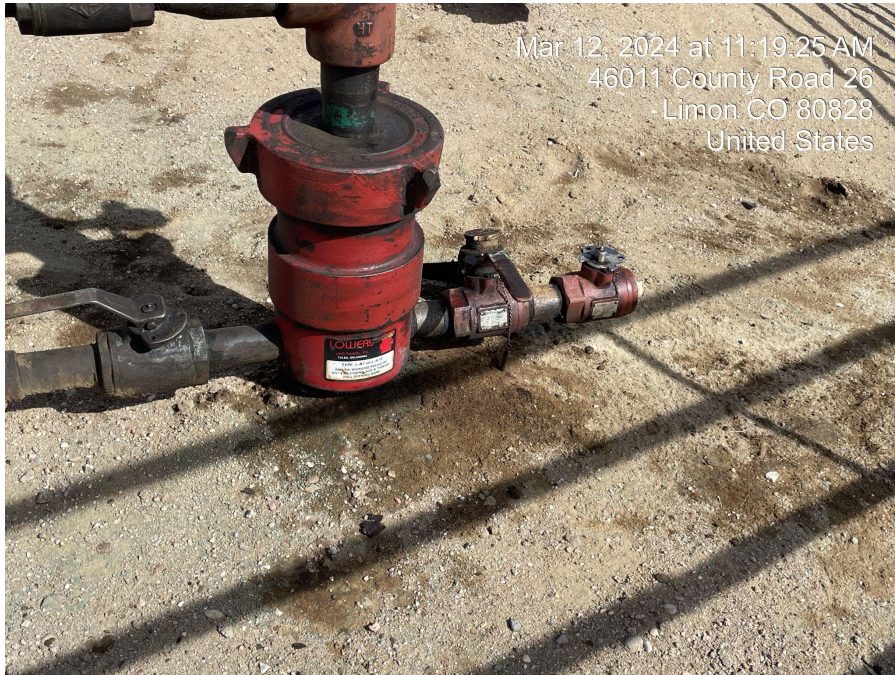
Photo 3. Photo taken facing northeast of stained soil around wellhead.
