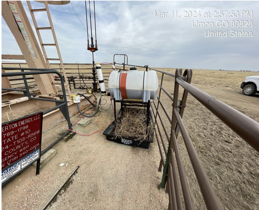
Photo 3. Photo taken facing west of secondary containment without wildlife protection.
