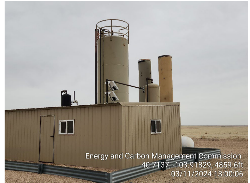
Photo 10 – Heater Treater and ECDs
