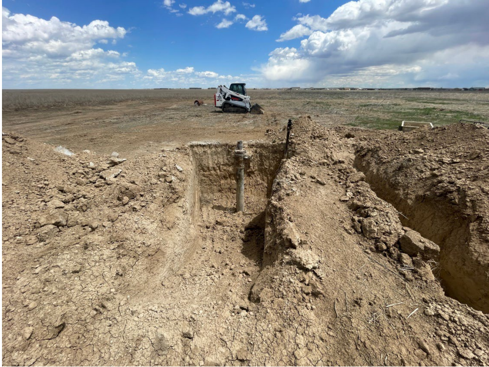
WH2) wellhead excavation with flowline rise, with concrete spillage in foreground - facing west
