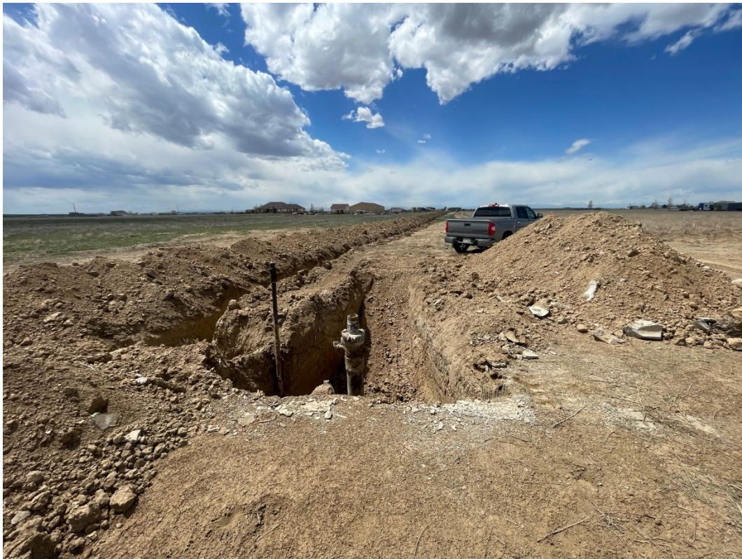
WH2) wellhead excavation with flowline rise, with concrete spillage in foreground - facing west
