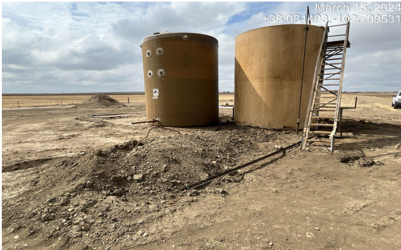
Photo 5. Facing west toward the tank battery which had been significantly remodified and requires secondary containment per Rule 603.o. There is also no labeling of the crude oil tank at the right side of the photo. The produced water tank is labeled at the left tank.
