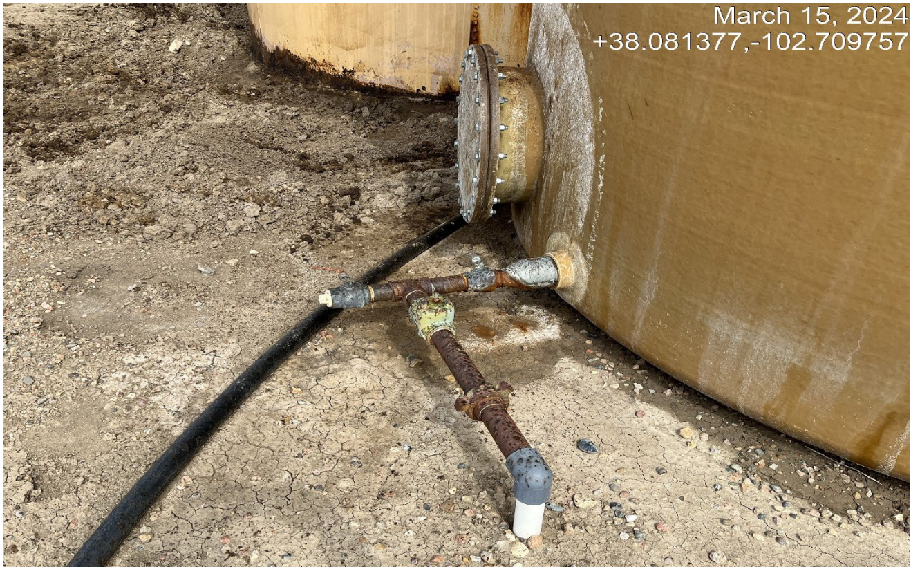
Photo 4. Closer view at the tanks. It appear the produce water tank has a dripping leak. The oily soils around the crude oil tank have not been properly cleaned up.
