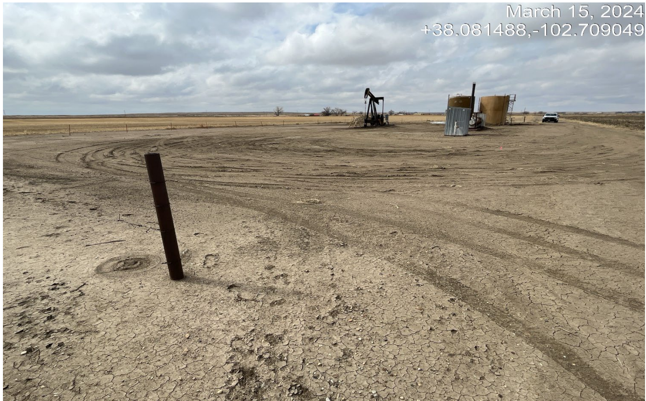
Photo 10. Facing southwest at the location. Unused areas of the location are not reclaimed. Fence is only up on the sides and does not prevent livestock entry.
