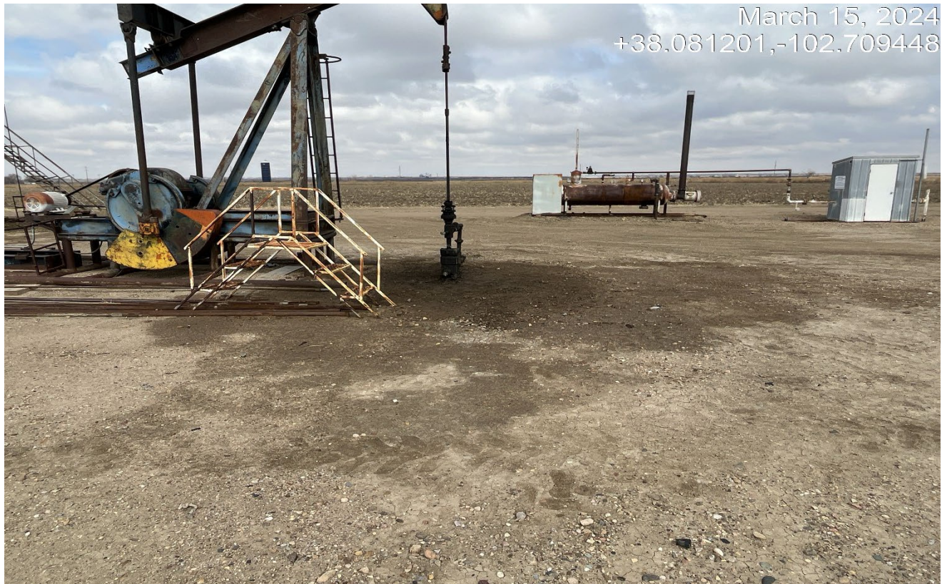
Photo 7. Facing north toward the wellhead. There is oil that has leak and sprayed out of the wellhead that needs to be cleaned up. Previous corrective action has not been completed.
