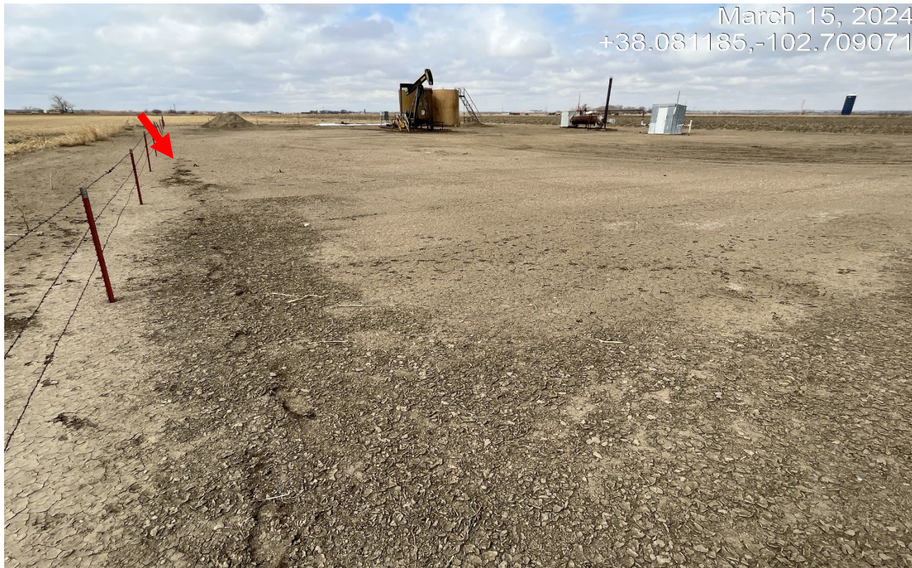
Photo 9. Facing west at the south side of the location. Red arrow points to the unmarked guyline anchor. Unused areas of the location are not reclaimed.
