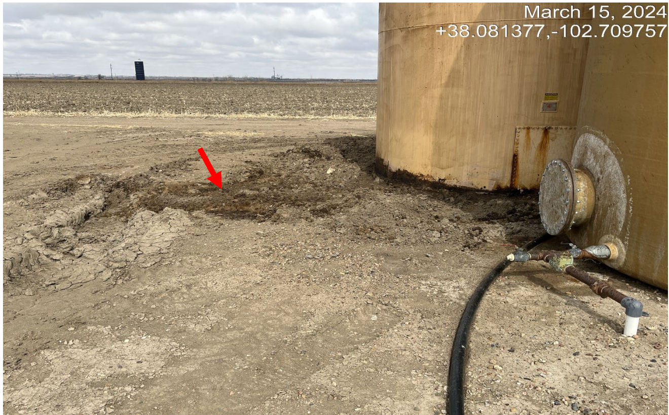
Photo 3. Facing northeast toward the tank battery where leak was previously observed. It appears the impacted material was partially scrapped away however there is still dark oily soil still evident around the tanks that extends out shown by red arrow.
