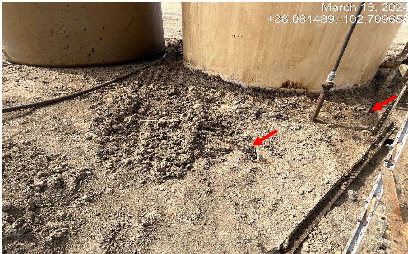
Photo 6. Facing west toward the tank battery where leak was previously observed. It appears the impacted material was partially scrapped away however there is still dark oily soil still evident around the tanks. Tanks will need to be removed for proper clean up.
