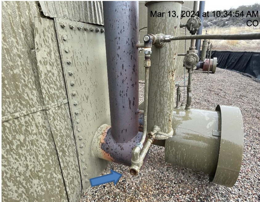
Photo # 9626 PRV vent line on tank burner terminates in an unsafe manner/does not comply with CECMC pressure safety device rules & general safety rules.
