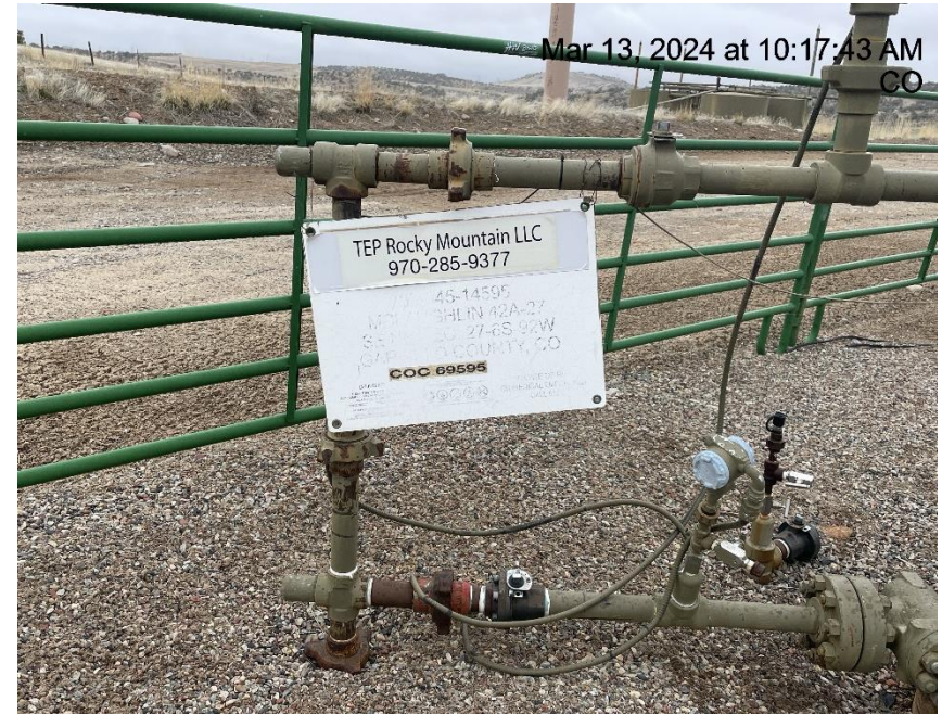
Photo # 9627 42A-27 wellhead sign faded & illegible
